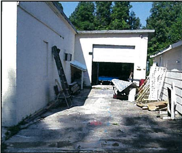
Looking Northeast between the back of the store front (on the right) and shop (on the left) – Note: DPT-05 marking in pink
