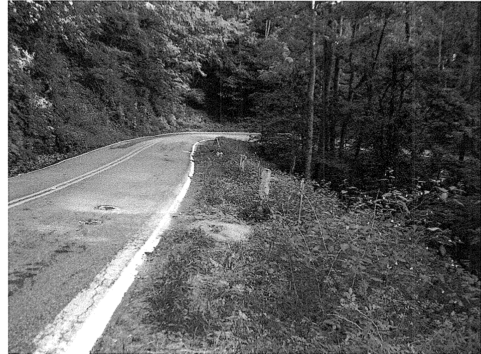
Photograph 1 – View Along Retaining Wall at Site 4 Looking Upstation
