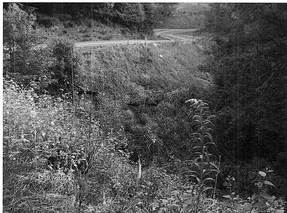
Photograph 2 – View Along Retaining Wall 2, Site 1 Looking Upstation
