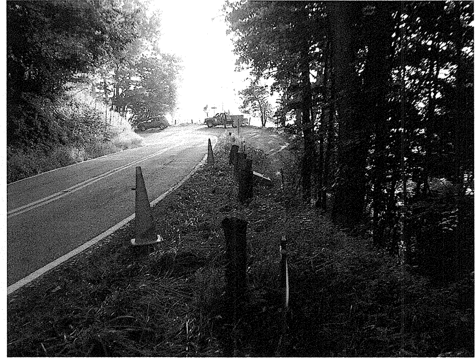
Photograph 1 – View Along Retaining Wall 1, Site 5 Looking Upstation
