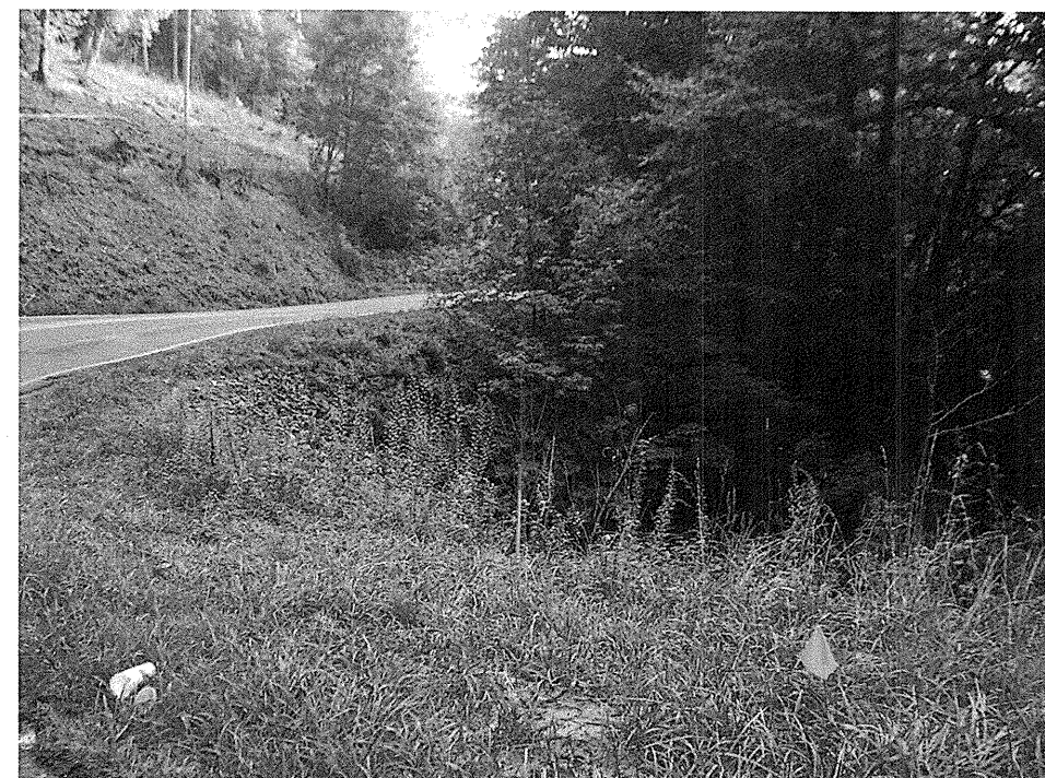
Photograph 3 – View Along Retaining Wall 3, Site 1 Looking Upstation
