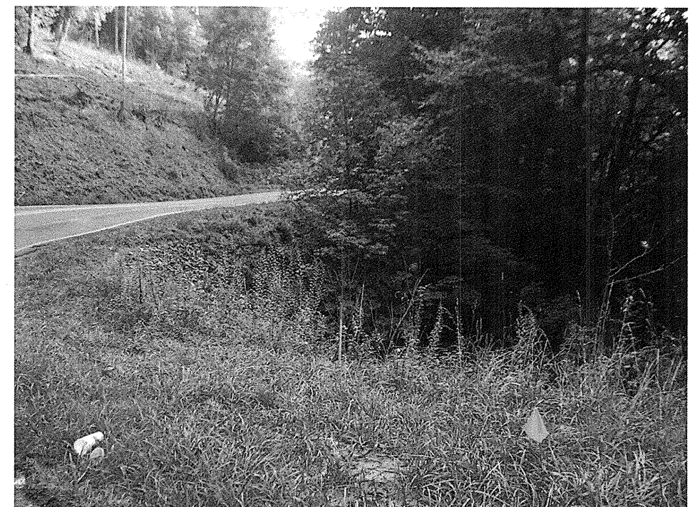
Photograph 3 – View Along Retaining Wall 3, Site 1 Looking Upstation
