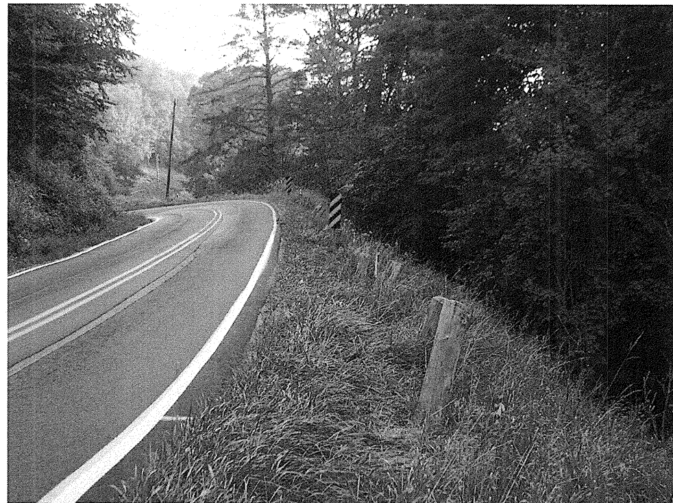
Photograph 1 – View Along Retaining Wall 1, Site 1 Looking Upstation
