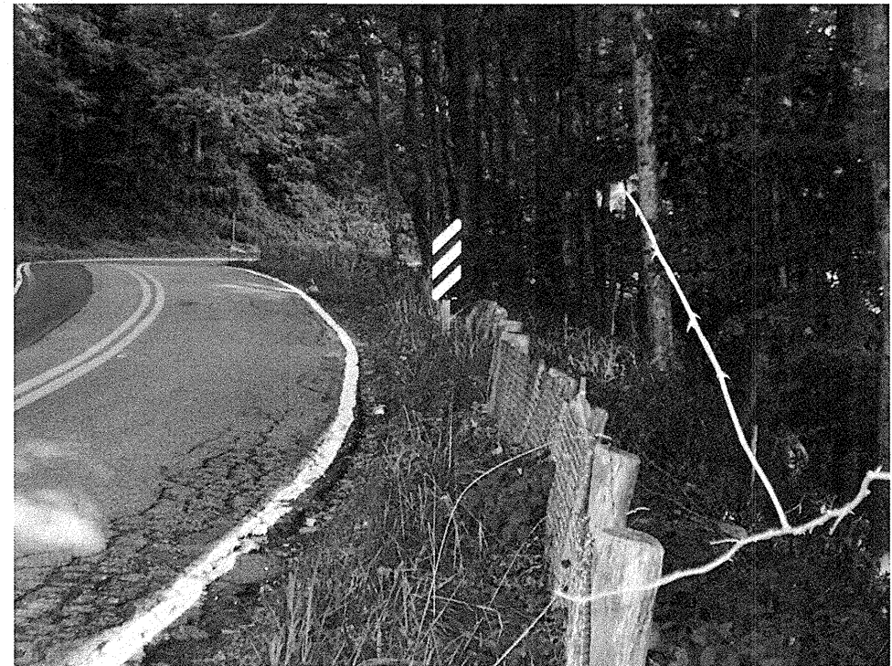
Photograph 2 – View Along Retaining Wall 2, Site 5 Looking Upstation
