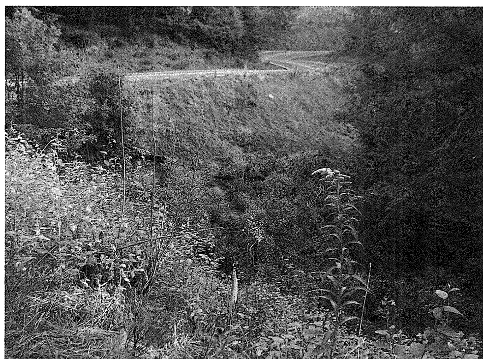
Photograph 2 – View Along Retaining Wall 2, Site 1 Looking Upstation
