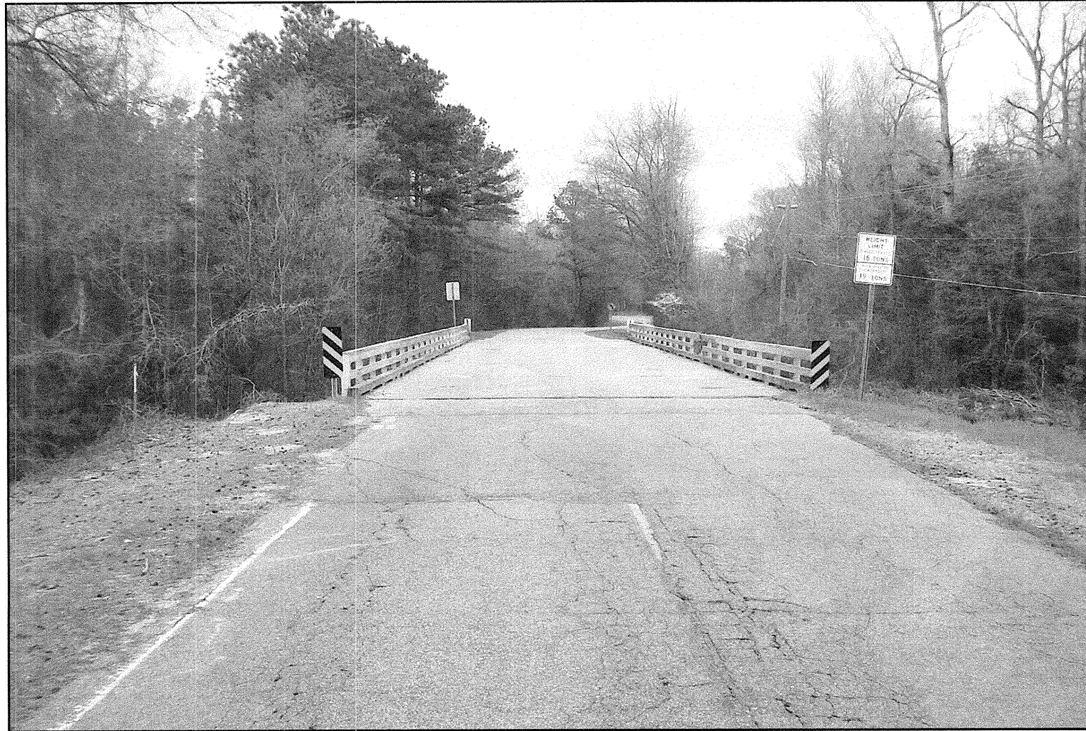
OVERVIEW OF EXISTING BRIDGE, LOOKING NORTH (UPSTATION) FROM NEAR END BENT 1.
