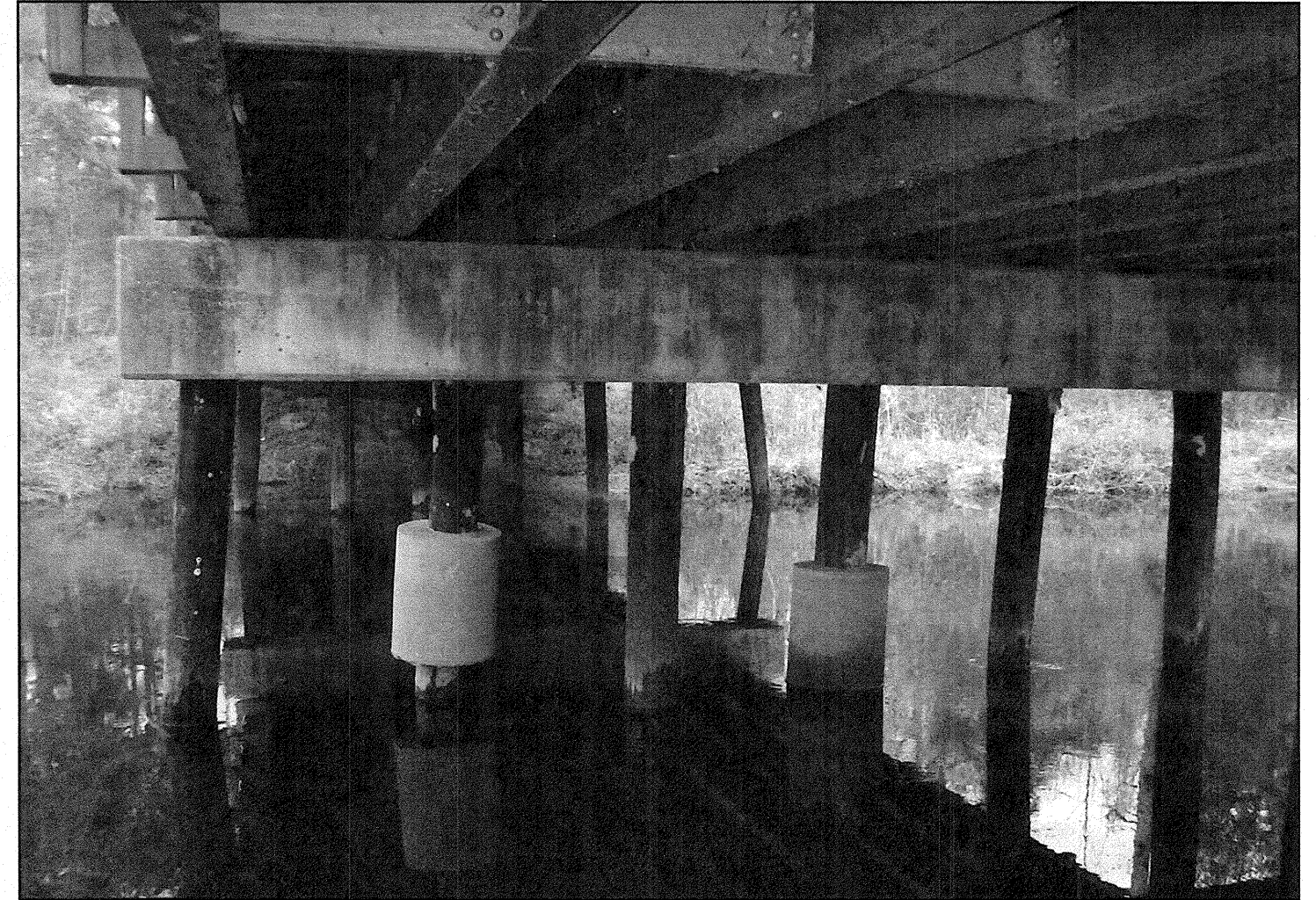
EXISTING BRIDGE LOOKING NORTH (UPSTATION) AT BENT 1 AND BENT 2.
