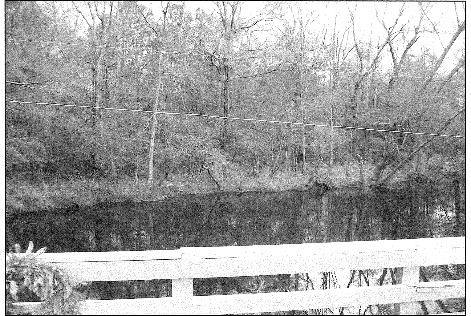
LOOKING EAST AT LITTLE RIVER (DOWNSTREAM) FROM EXISTING BRIDGE.
