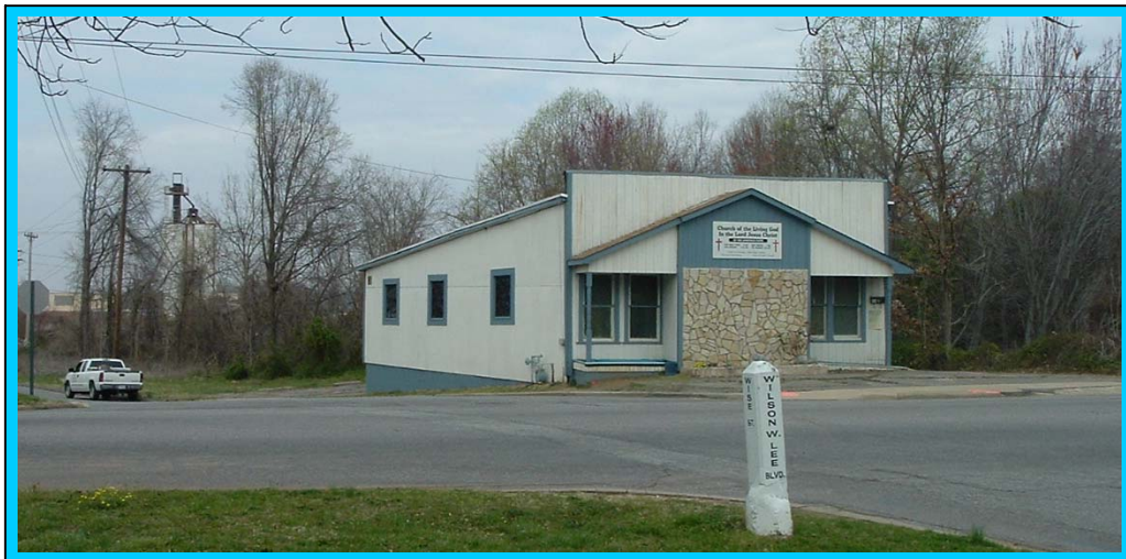
The photo shows a portion of the geophysical survey area located at the Church of the Living God site. The photo is viewed in a westerly direction.
