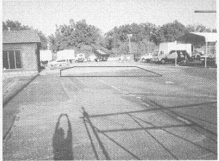
Photograph 4: View of former UST tank pit location (Center of photo).
