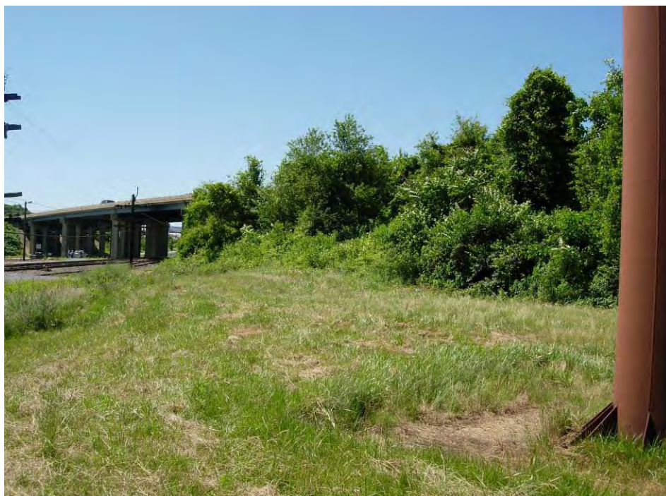
Photo 10 – View of north side of Route 52 bridge looking south.
