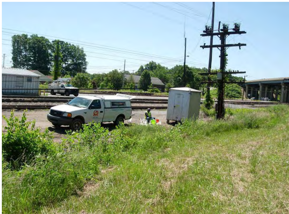
Photo 9 – View of temporary decontamination station.
