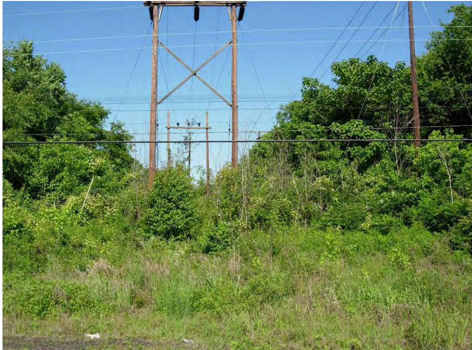
Photo 3 – View of power transmission right-of-way looking west.
