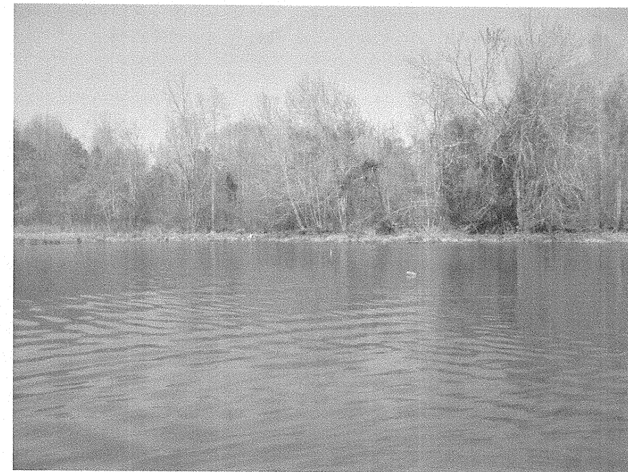
Photograph No. 7: This photograph was taken from the left side of the -I9FLY- alignment, looking north, across proposed End Bent No. 2.
