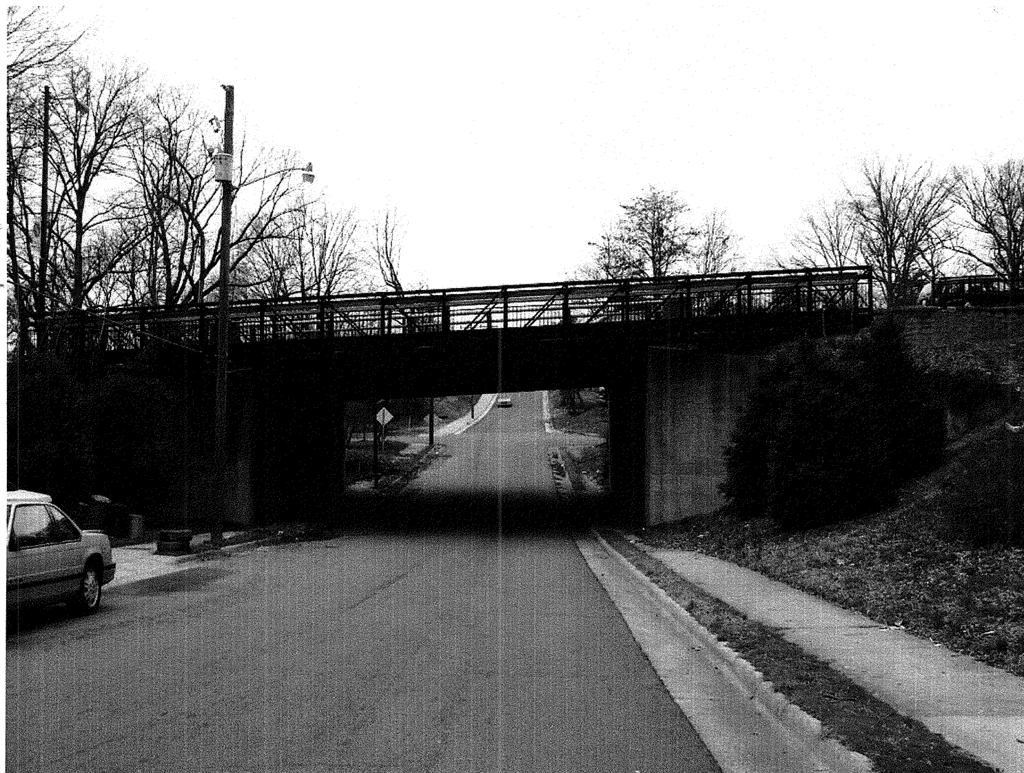
B-4745 EAST FACE OF BRIDGE
