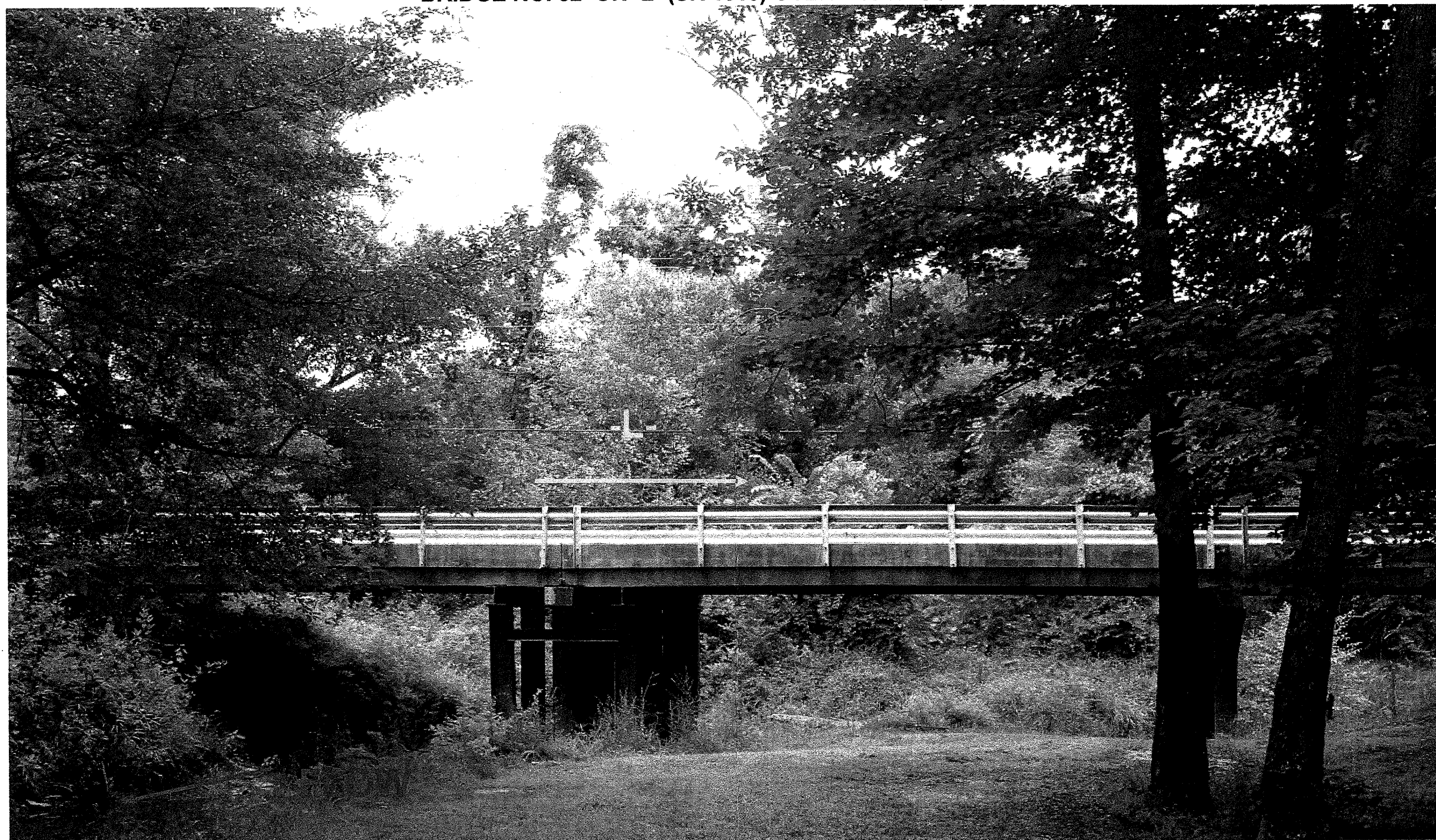
LOOKING NORTHEAST TOWARD BENT 1
