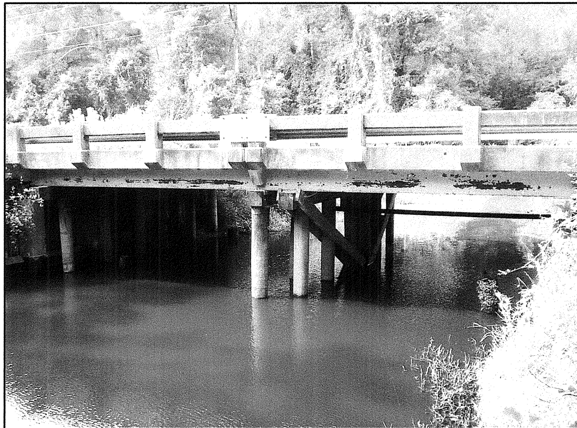
BRIDGE 9 FACING DOWNSTREAM (SOUTHWEST)
