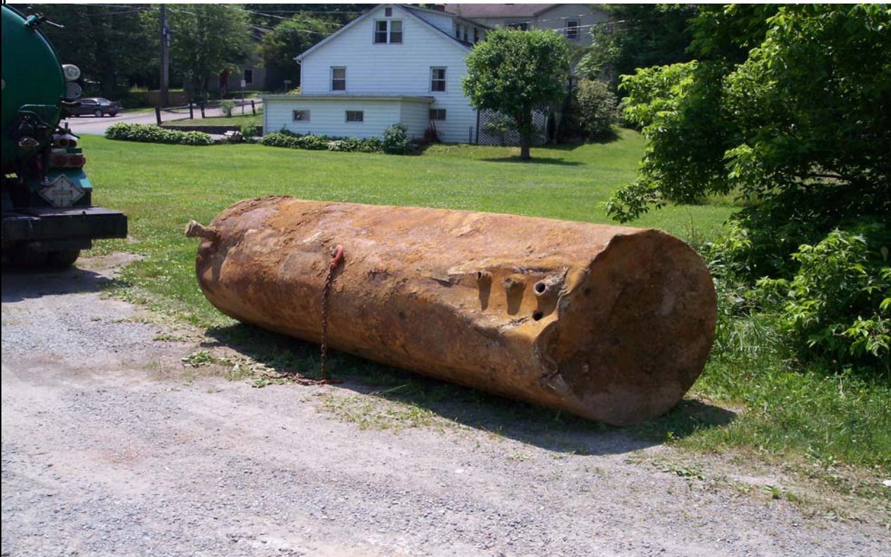
Photograph 2: Removed UST from Parcel 28.
