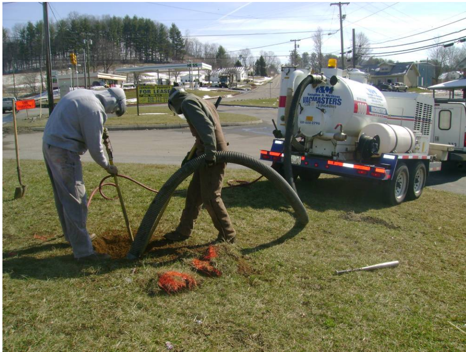
Start of air excavation with Vacmasters 1000 unit
