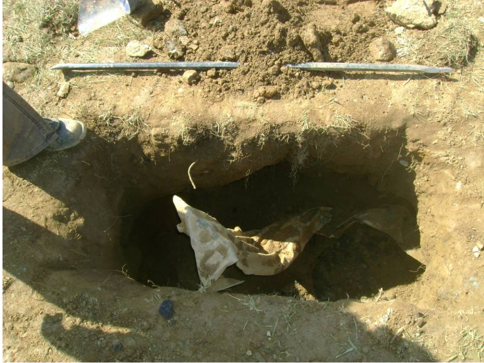
End of air excavation
