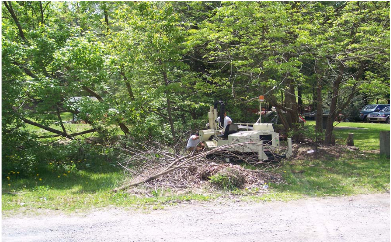
Photograph 6: Geoprobe temporary well installation at P28-17.
