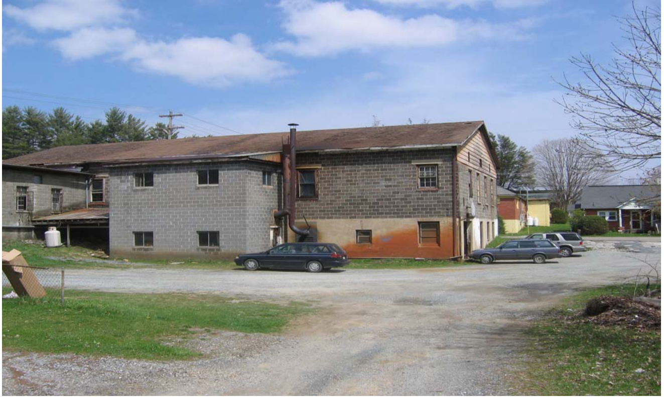
Photograph 1: Parcel 28 facing east at the back of the dry cleaners.
