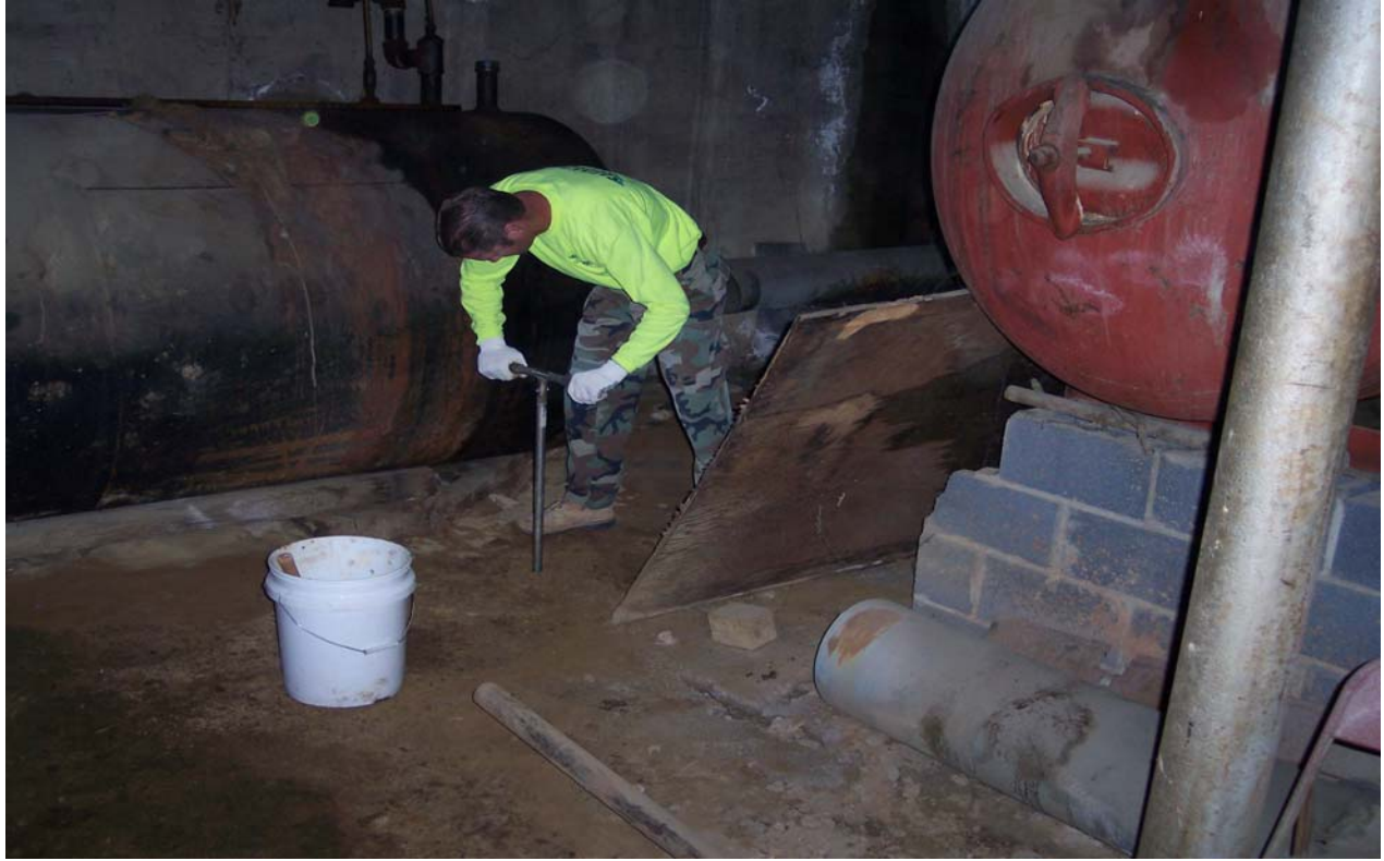
Photograph 5: Hand auger sampling next to the current AST in basement.
