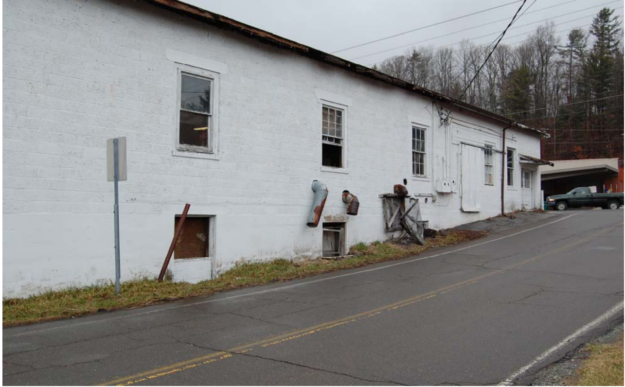
Photograph 3: Parcel 28 looking northwest along the east wall of Trailway dry cleaners.
