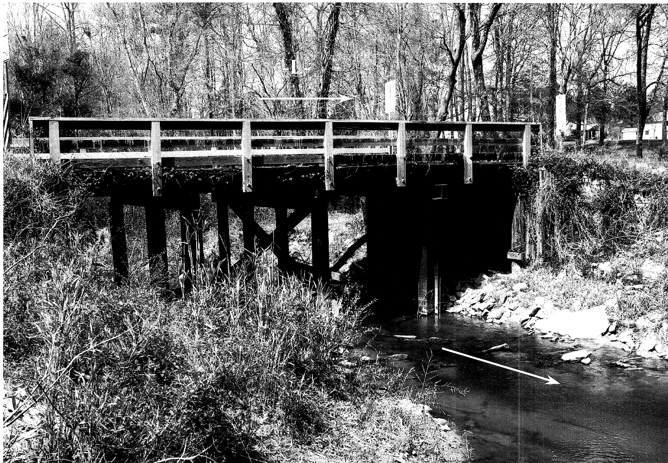
Bridge No. 151 on -L- (SR 1146) over Camping Creek
