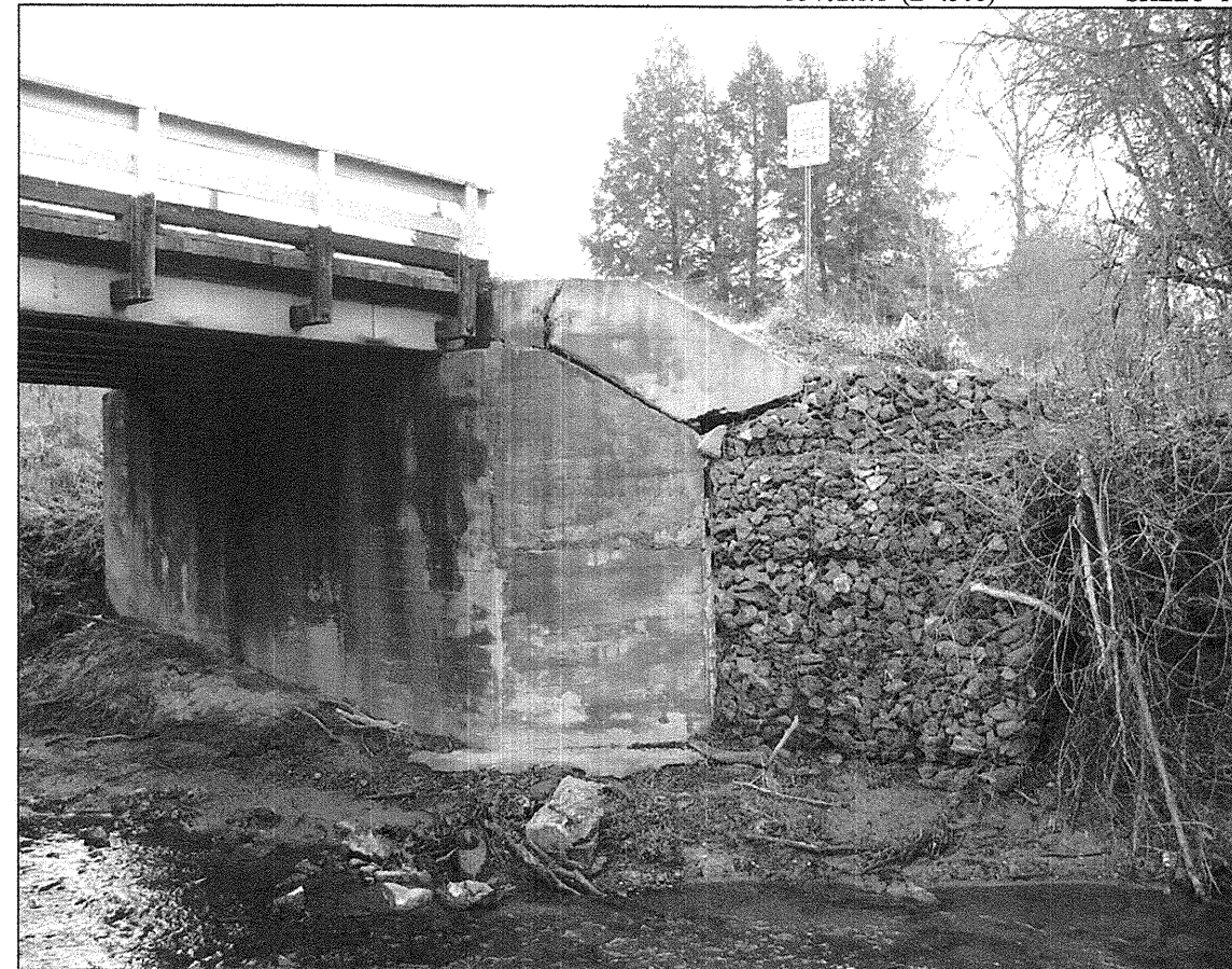
Photos 4-6: Looking at damaged wing wall repaired with Gabion baskets.
