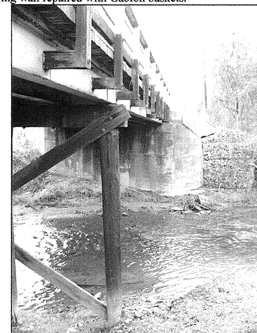
Photos 4-6: Looking at damaged wing wall repaired with Gabion baskets.
