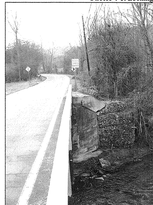
Photos 4-6: Looking at damaged wing wall repaired with Gabion baskets.
