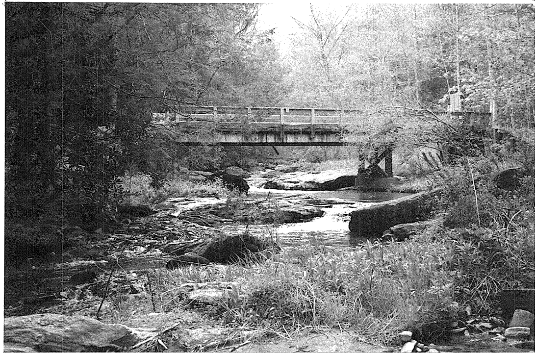
Figure 1. Bridge 70, looking upstream.
