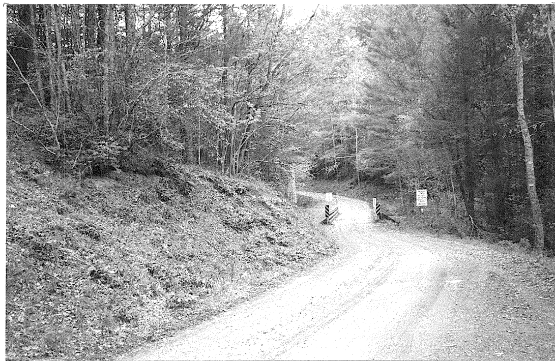
Figure 2. Looking forward from Station 13+00.
