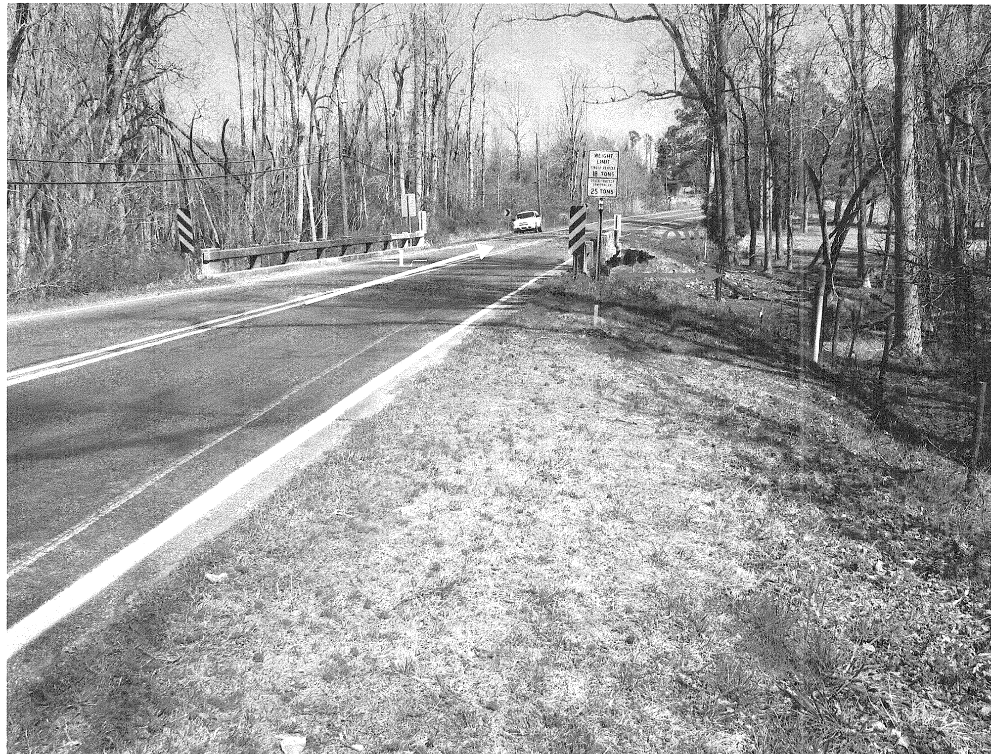
LOOKING NORTH TOWARDS END BENT 2
