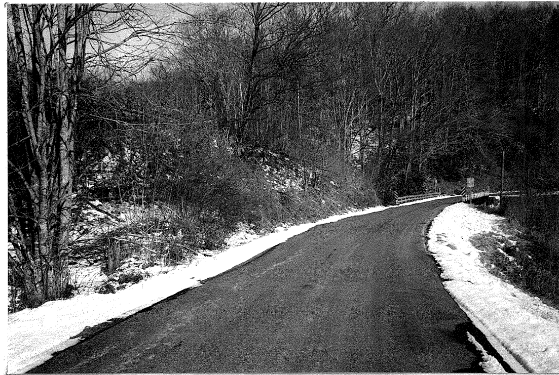
Fig. 3. View forward from Station 15+00
