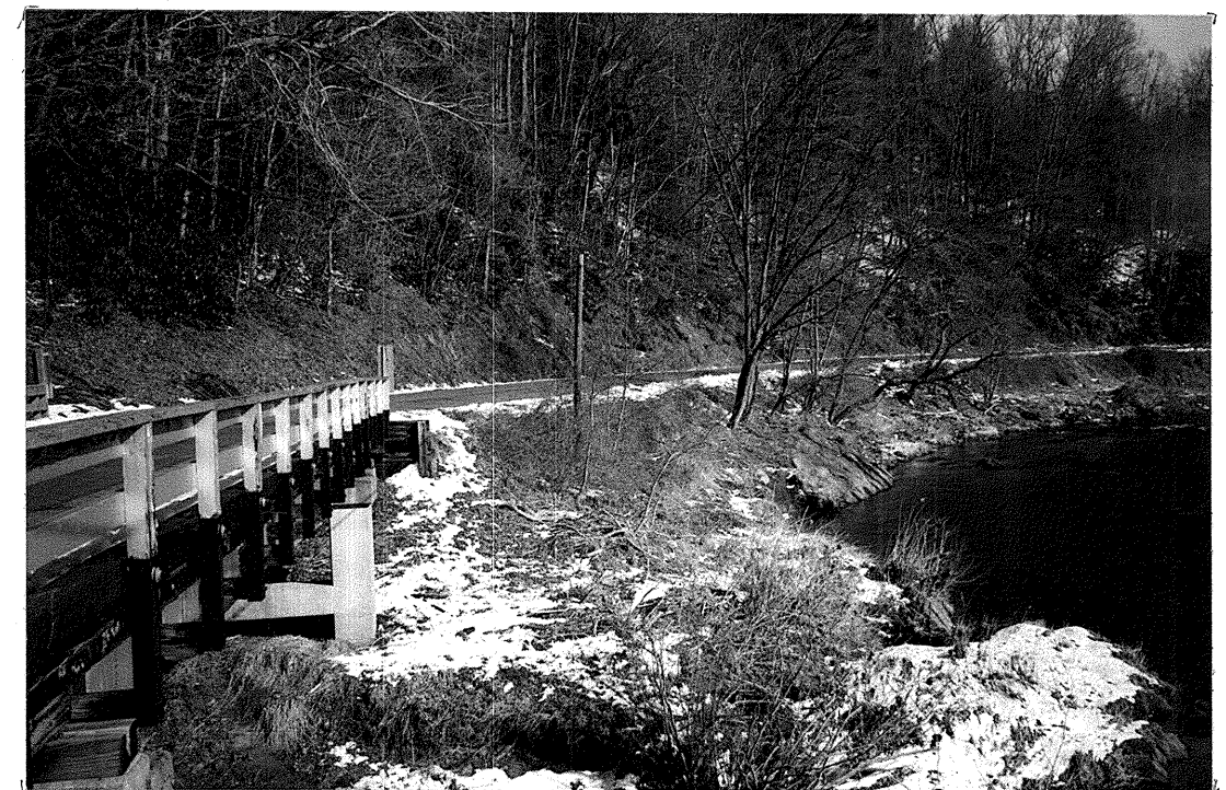
Fig. 6. View toward proposed wall site from Station 17+20
