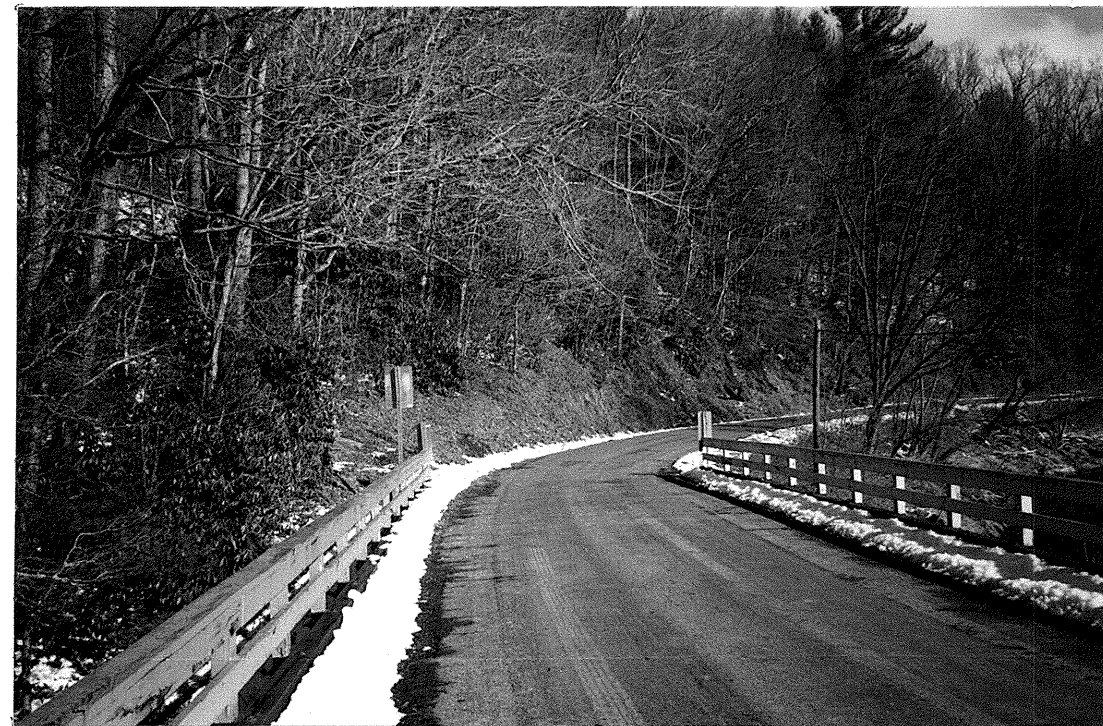
Fig. 4. View forward from Station 17+00
