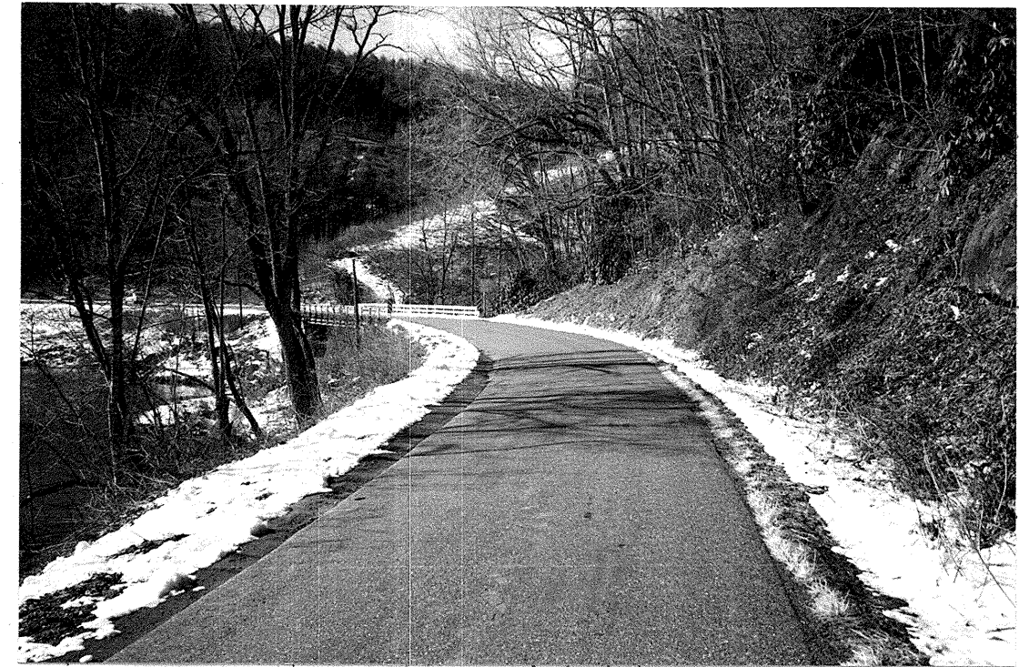
Fig. 5. View back from Station 20+50
