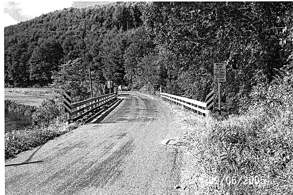
Photograph 2 – View of Bridge 85 Looking Downstation
