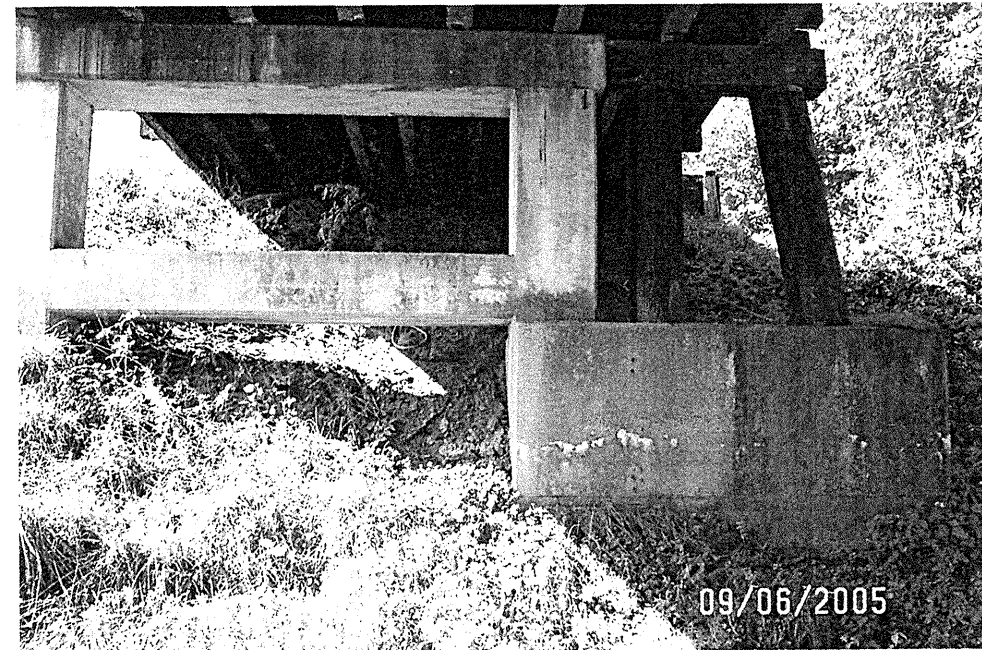
Photograph 6 – View of Interior Bent Support Structure at Bent-1
