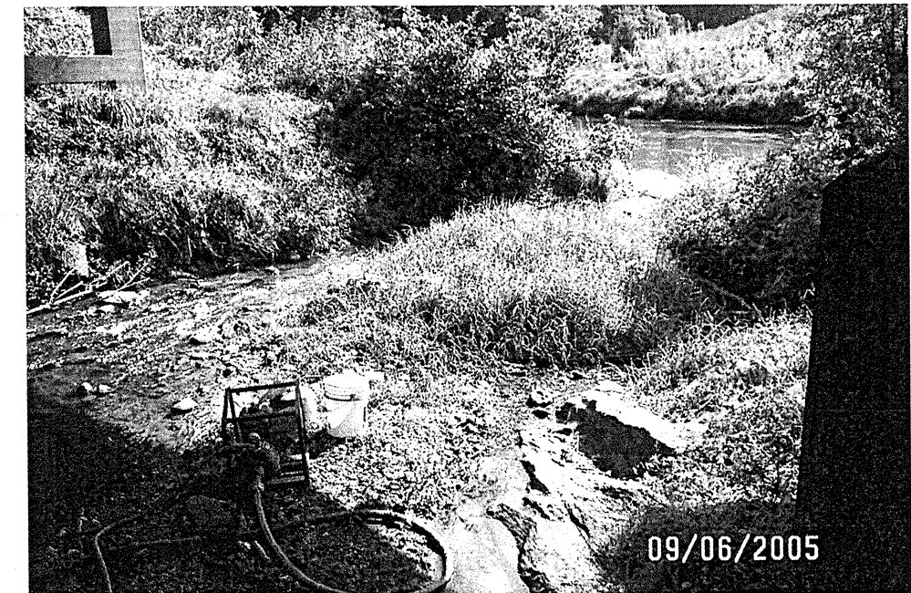
Photograph 4 – View Looking Downstream from Under Bridge
