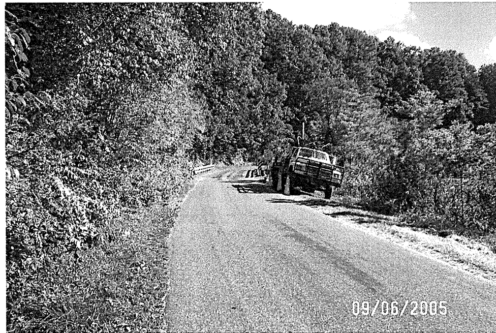
Photograph 1 – View of Bridge 85 Looking Upstation
