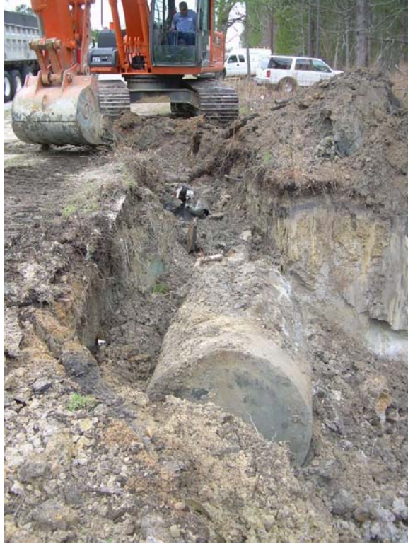
Photograph 1 - Tanks 1 & 2 uncovered.
