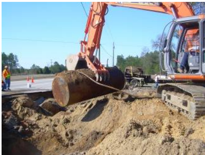
Photograph 6: Removing UST-4 and product line.
