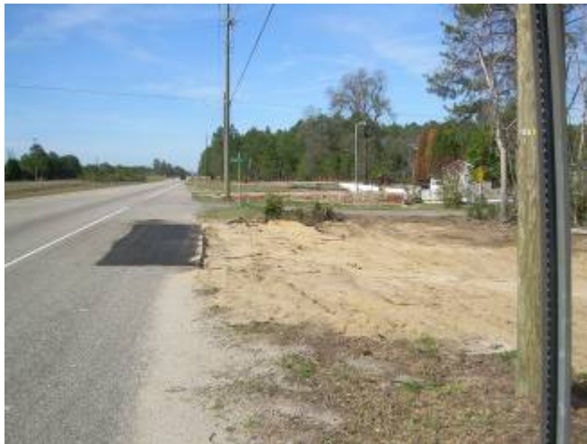
Photograph 9: following closure activities with repaired asphalt.
