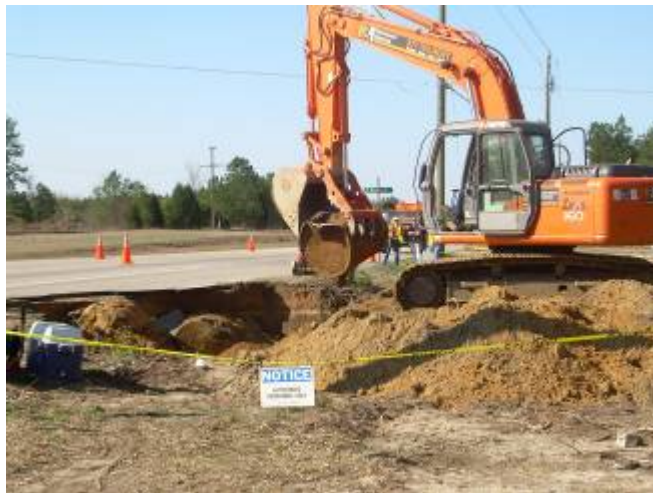
Photograph 3: Excavating UST 1
