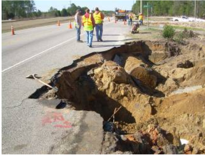
Photograph 7: UST 5 in place.
