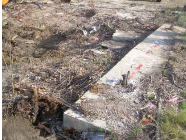
Photograph 8: Former dispenser island.
