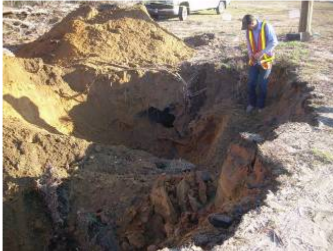
Photograph 4: UST 2 in place.
