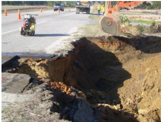
Photograph 2: Excavation looking westward.
