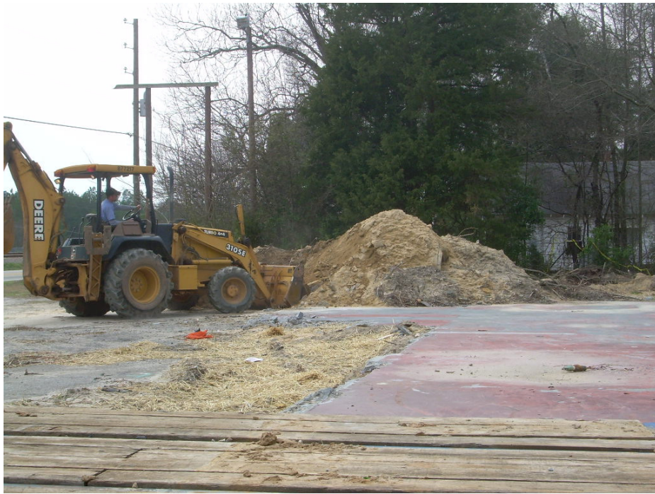
Loading Stockpiled Soil March 11, 2008; NCDOT Parcel 61
