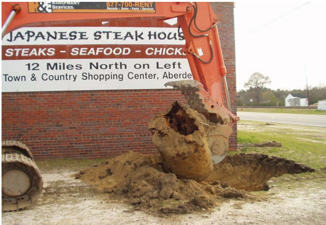
Photograph 1 – Tank removal
