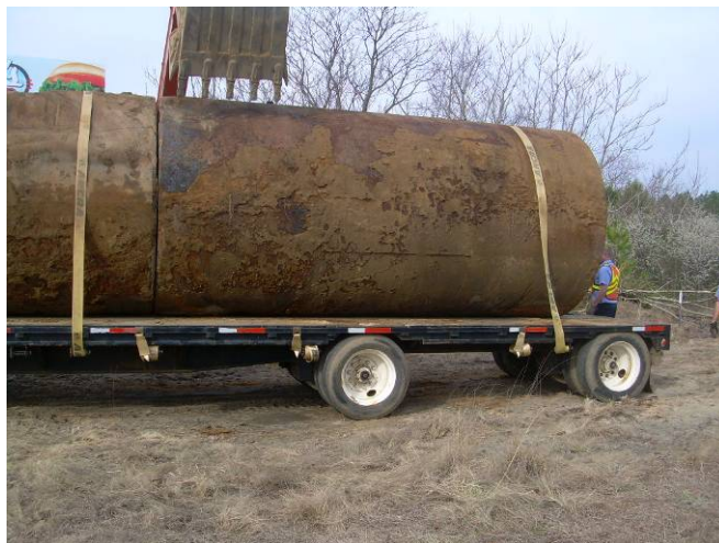
Two former USTs loaded on trucks.
