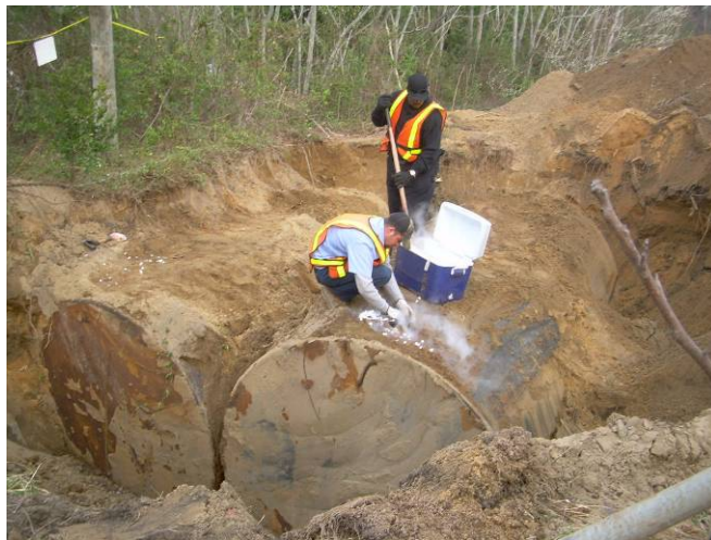
Preparing Tanks 1 and 2 for removal.
