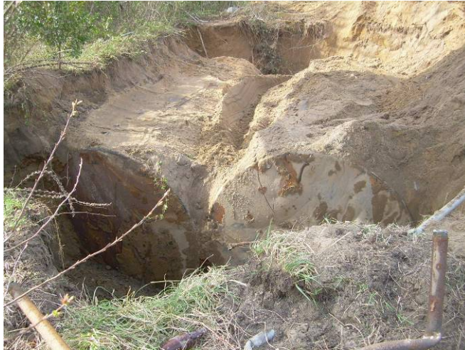
Parcel 21 tanks in place.
