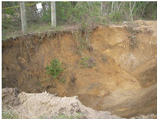
Excavation following tank removal.
