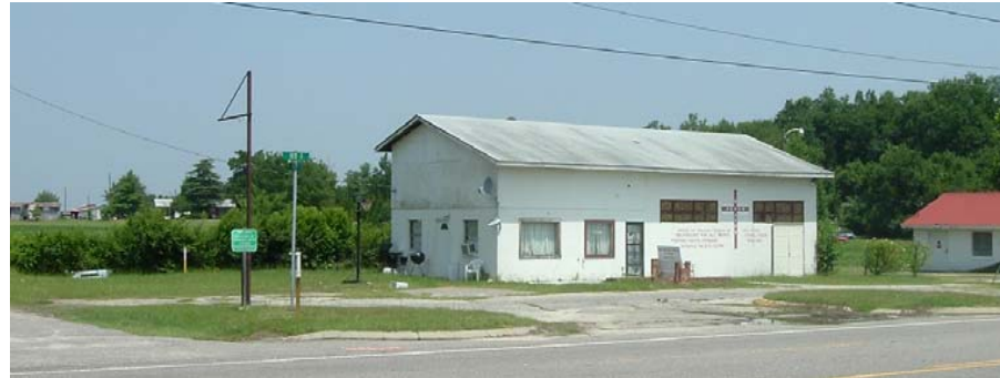
Parcel 51 - Church of Deliverance Property
