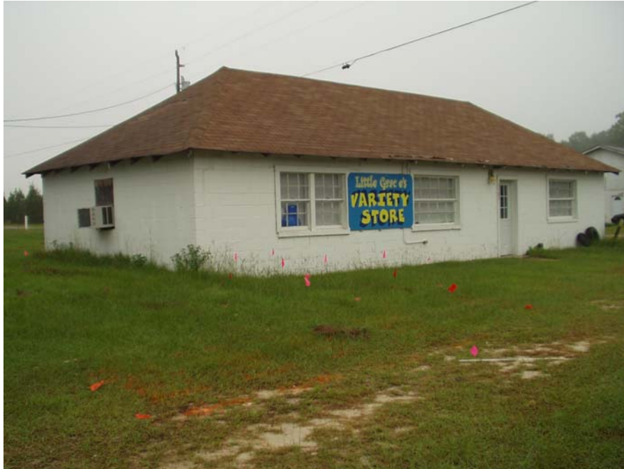
Photograph 1 – View from south to north from US Highway 1. Suspected UST locations in foreground.
