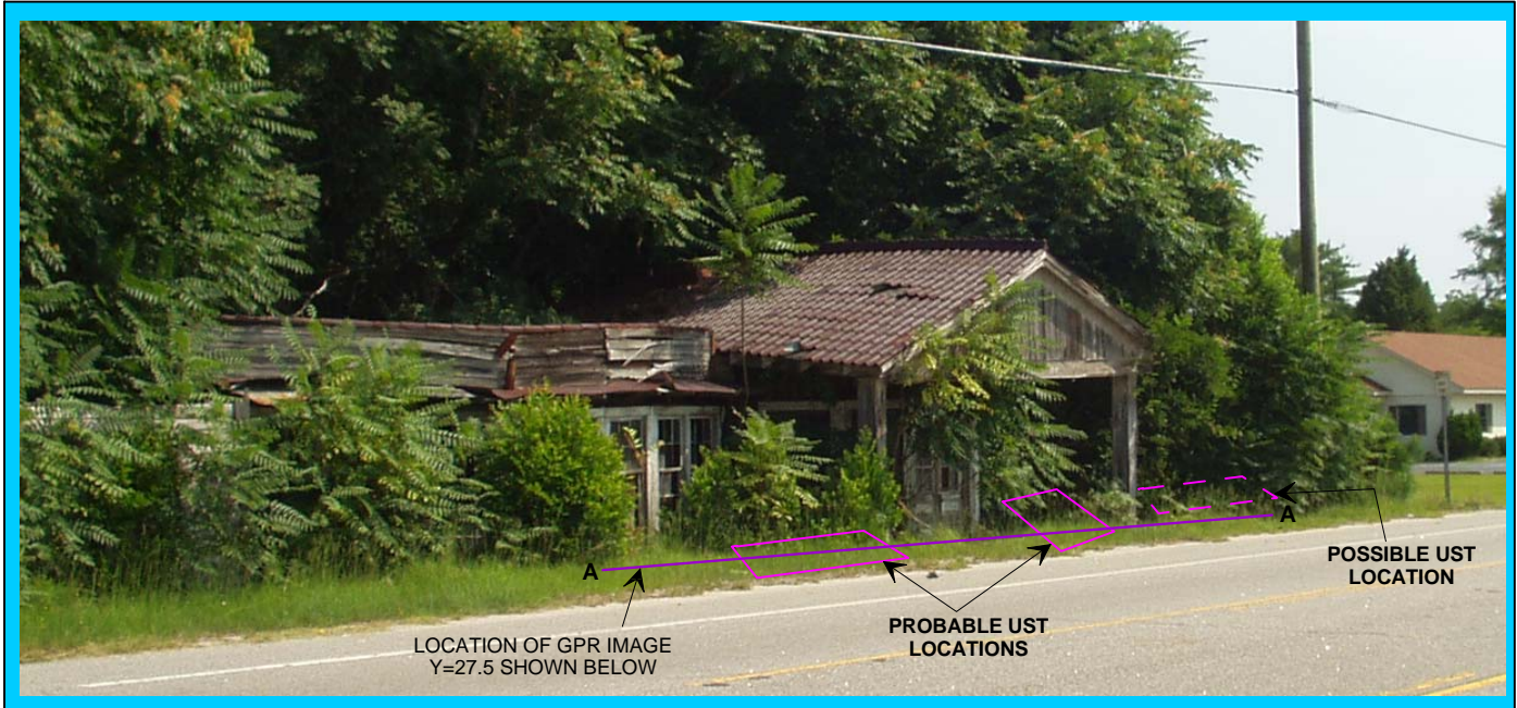
The photograph shows the locations of two probable USTs and one possible UST buried 1.5 to 2.0 feet below surface, as suggested by the geophysical results at Parcel 9.
