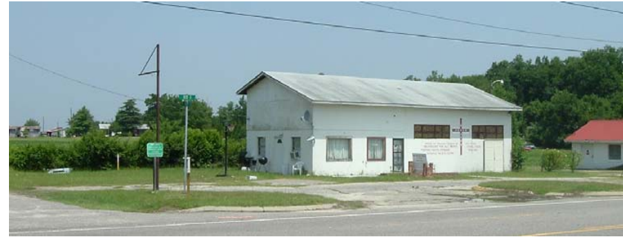
Parcel 51 - Church of Deliverance Property
