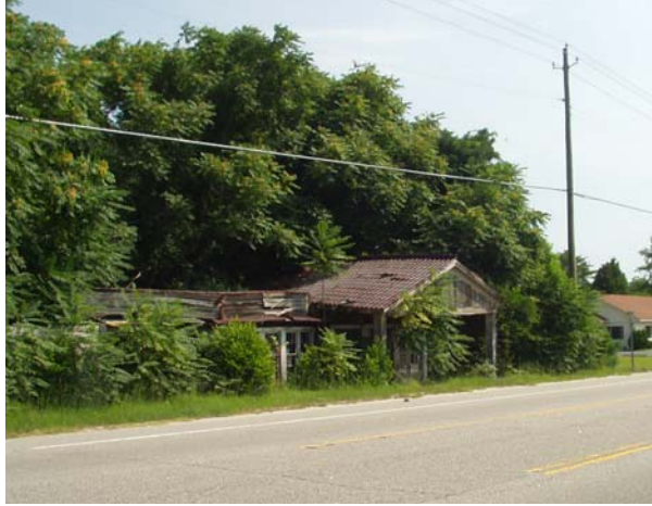
Photograph 1 – Looking north on US Highway 1 at Parcel 9.
