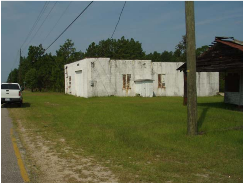
Photograph 1 – View of Parcel 6 from east to west along US Highway 1.
