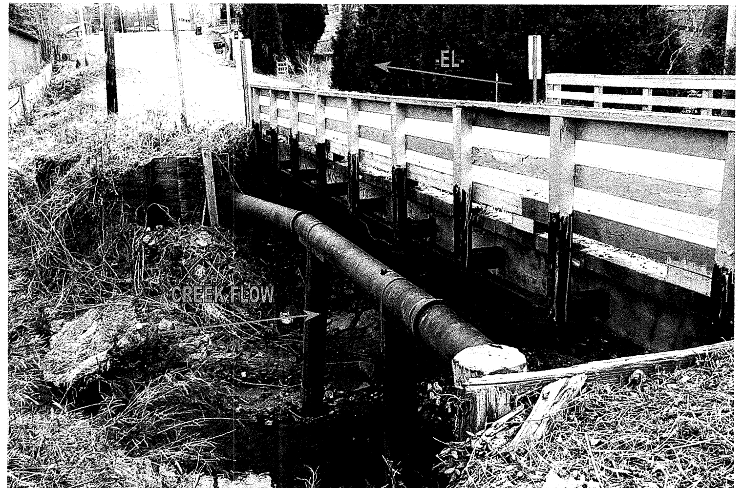
VIEW OF WATER PIPE
