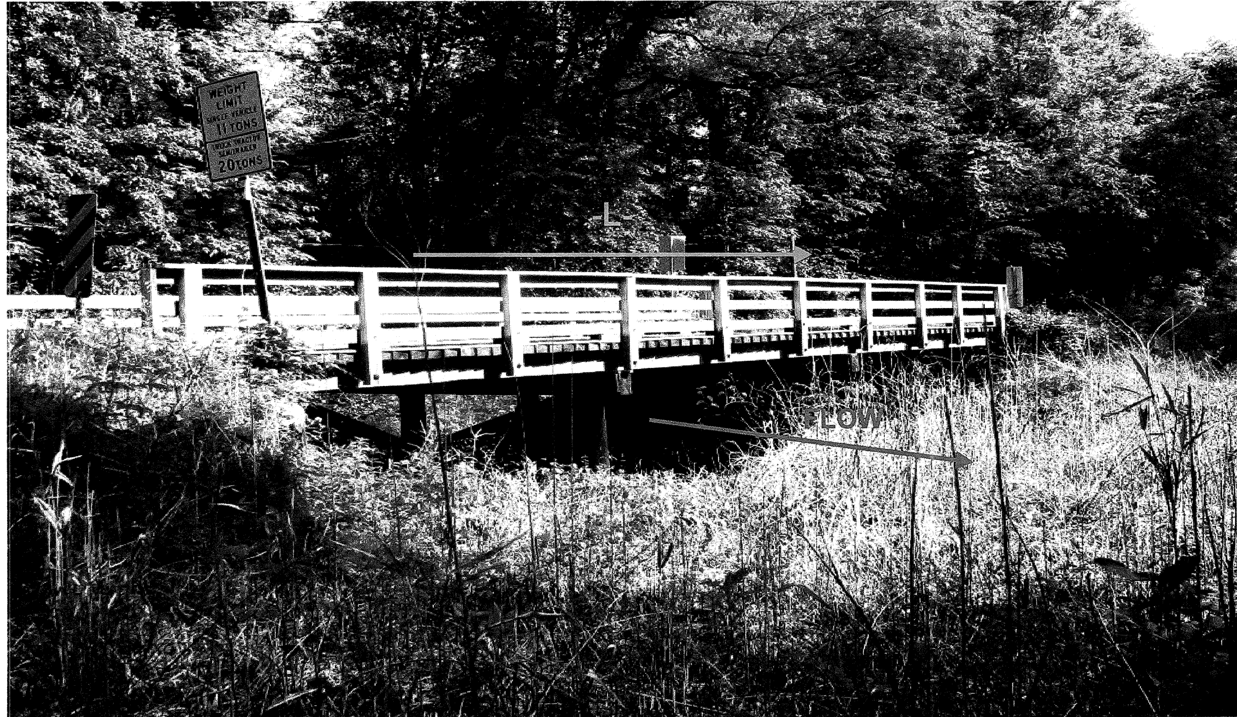
LOOKING NORTHWEST FROM EB1-B
