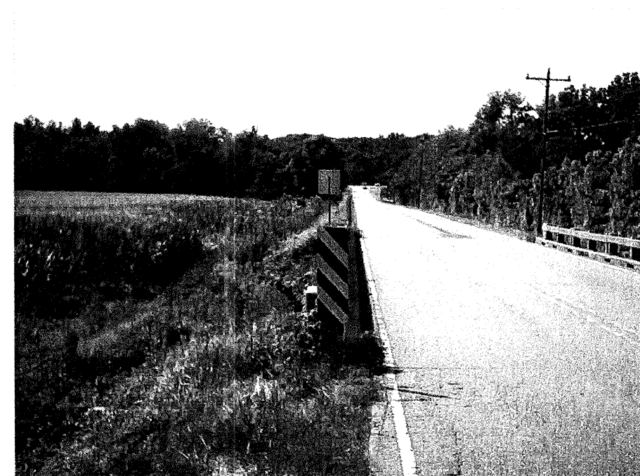
Photograph No. 8: This photograph was taken from the right side of the existing bridge, looking south.
