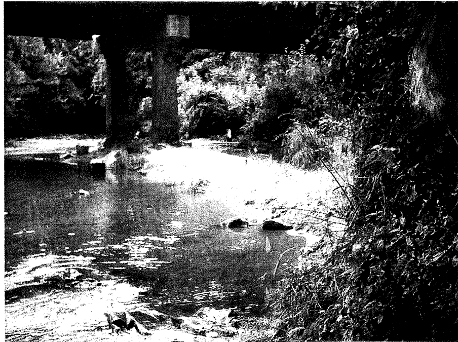
Photograph No. 5: This photograph was taken from the right side of the -L- alignment, looking west, across proposed Interior Bent No. 2.
