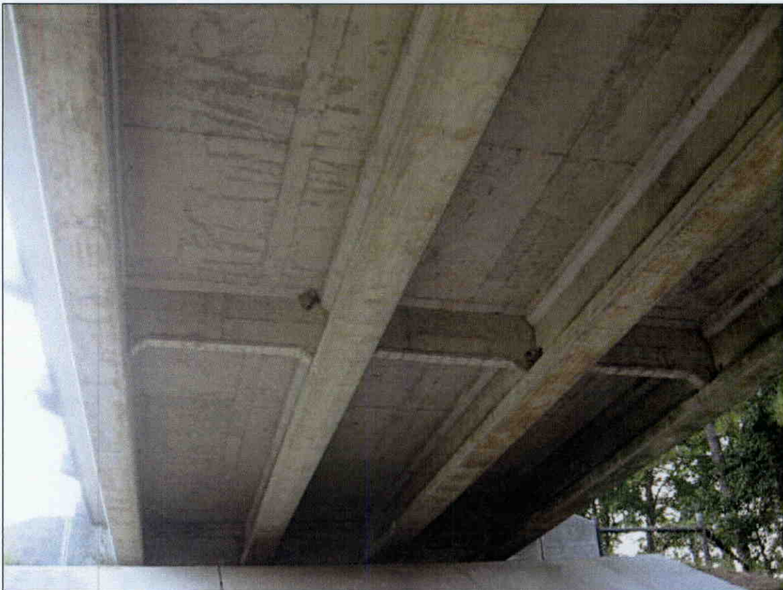
TYPICAL UNDERSIDE - SPAN 1
