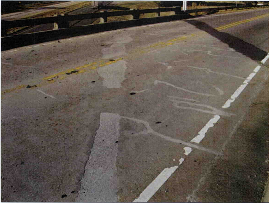
CONCRETE PATCHED AREAS ON DECK IN SPAN 5
