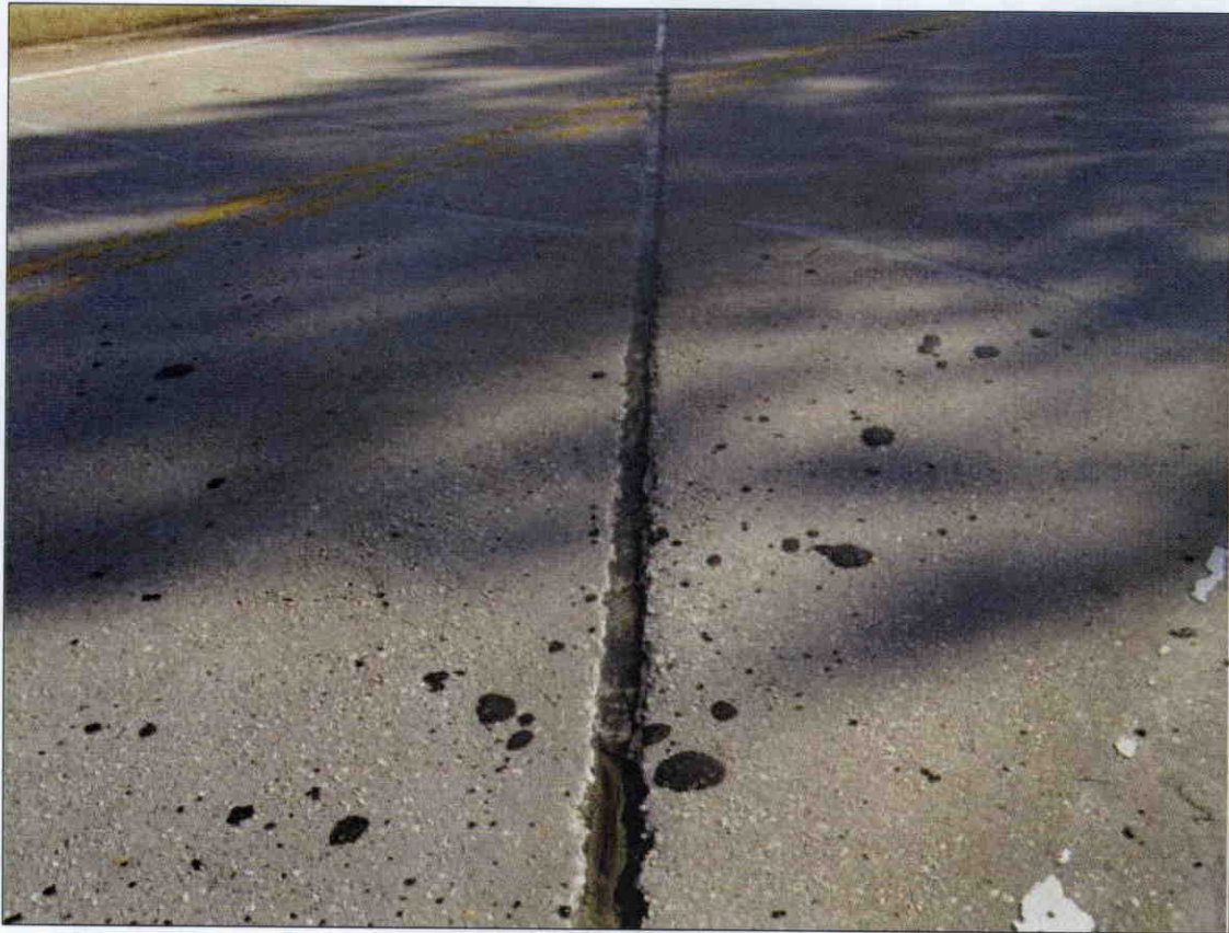
EXPANSION JOINT TYPICAL
