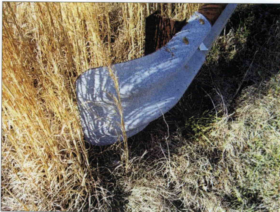
GUARDRAIL TERMINATOR SOUTHWEST CORNER
