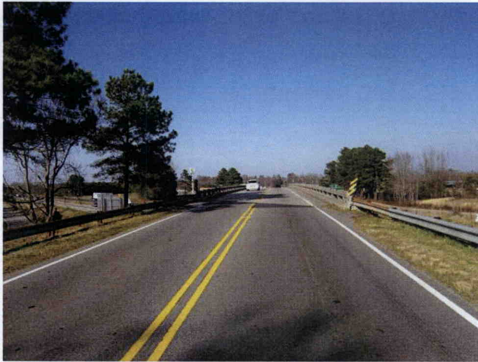
SOUTH APPROACH LOOKING NORTH
