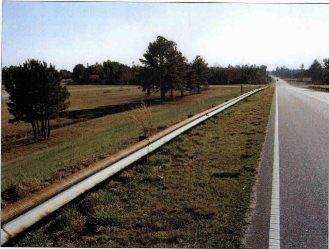
GUARDRAIL POST SPACING 12.25 FT. SOUTHEAST CORNER
