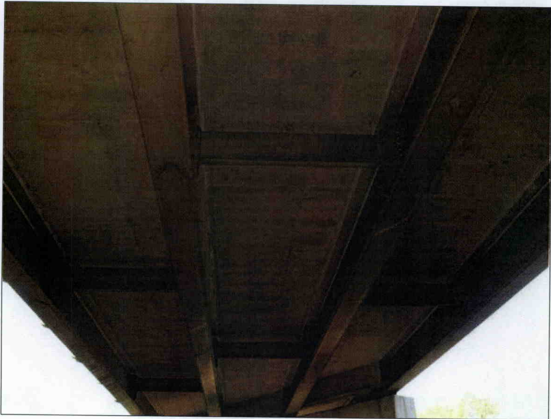
UNDERSIDE OF DECK
