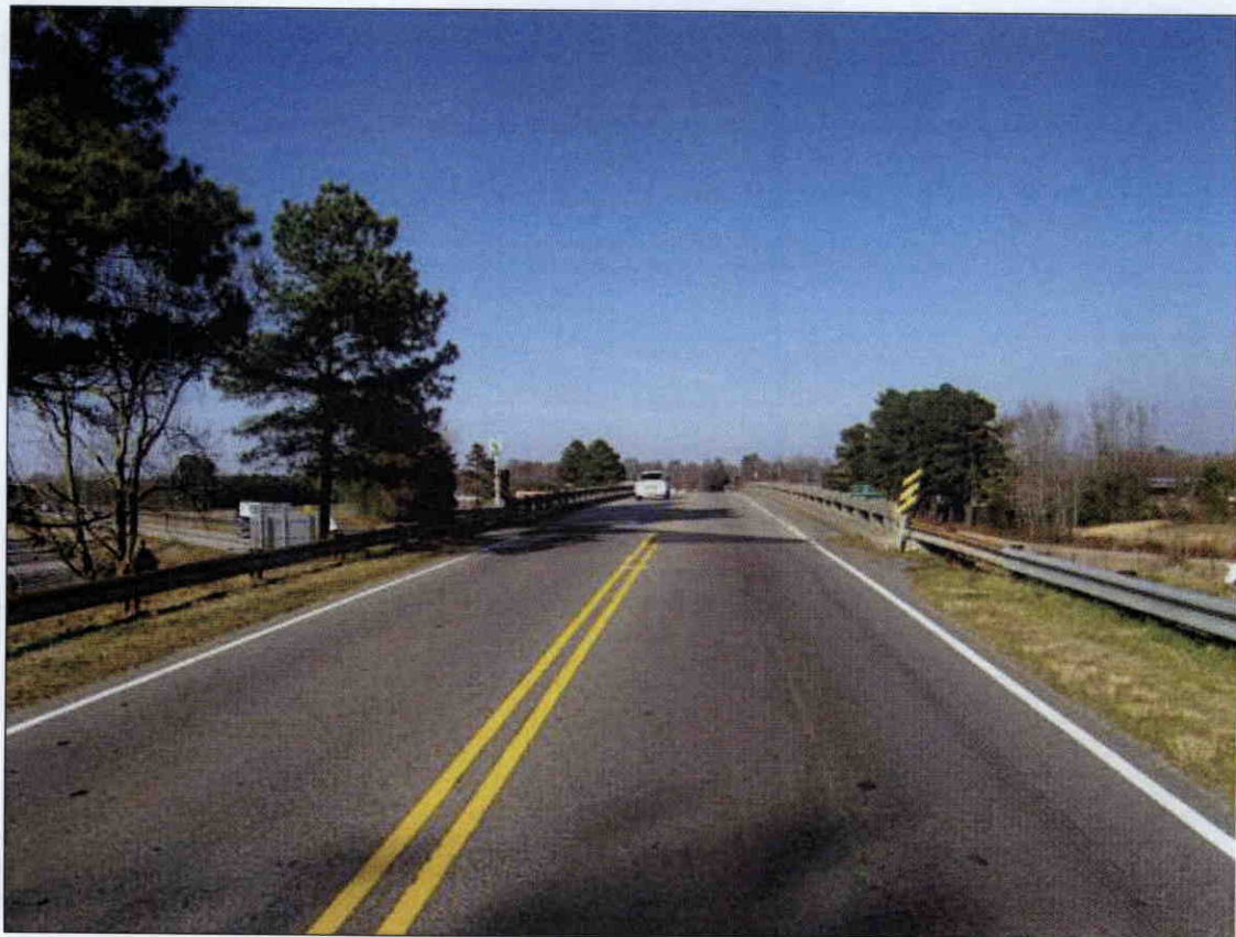
SOUTH APPROACH LOOKING NORTH
