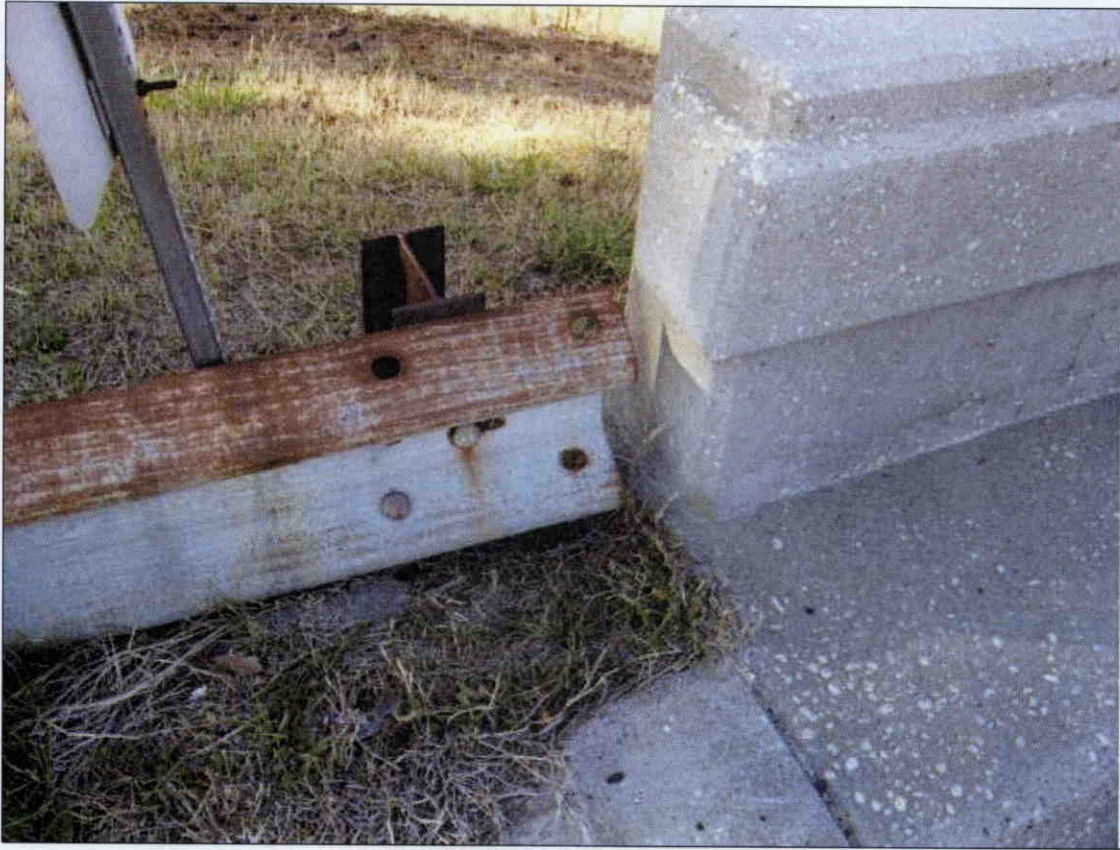
GUARDRAIL ATTACHMENT SOUTHWEST CORNER
