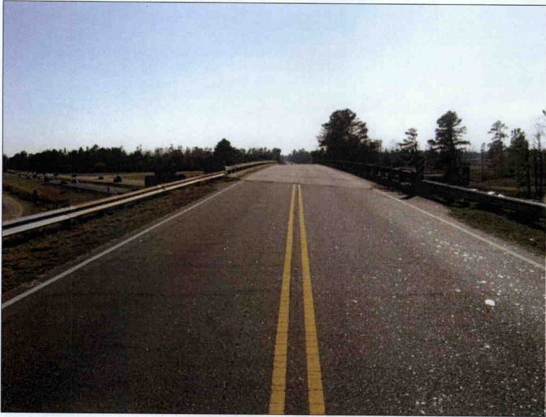
NORTH APPROACH LOOKING SOUTH
