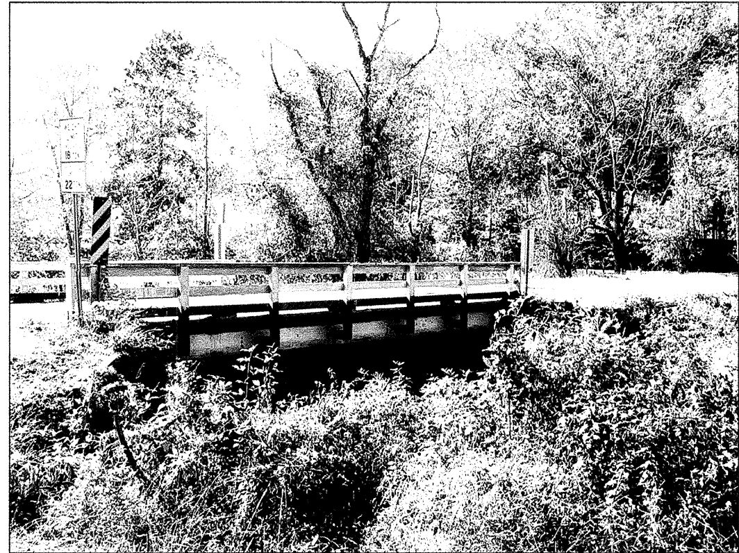
Photo 2: Looking South (Upstream) at bridge.
