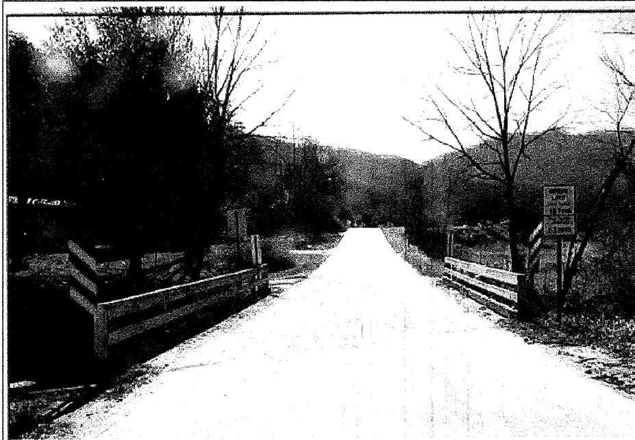
Photo 3: Looking East (Downstream) at -L-.
