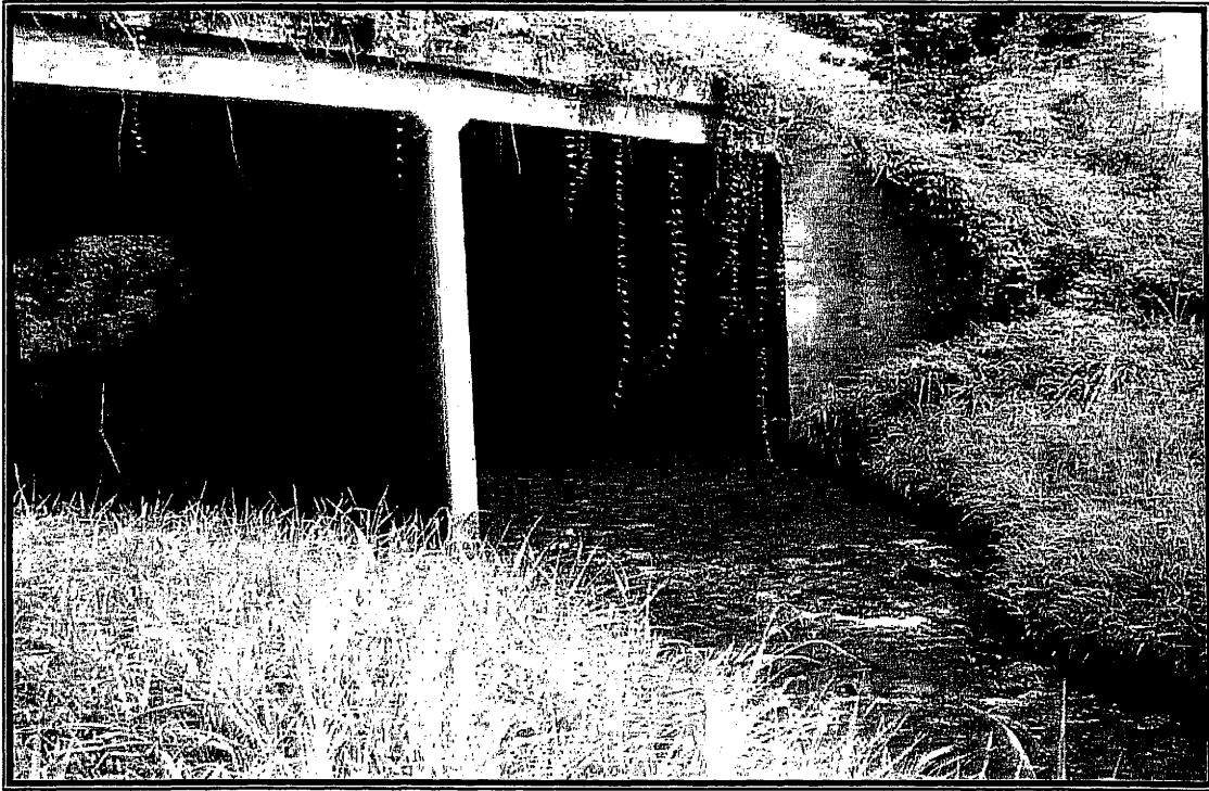
Site A: Roadway Station 19+80 UP
