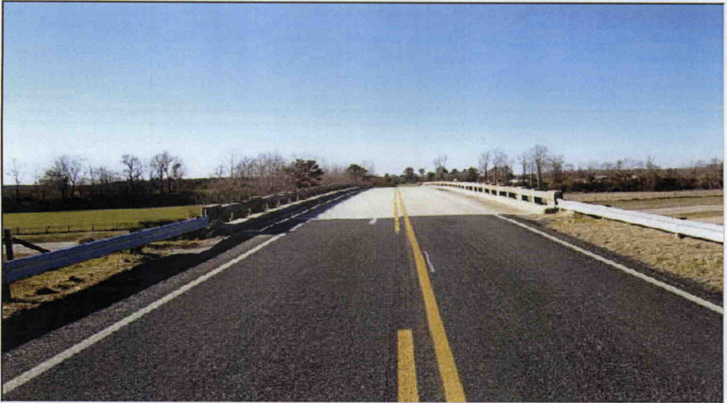
EAST APPROACH LOOKING WEST
