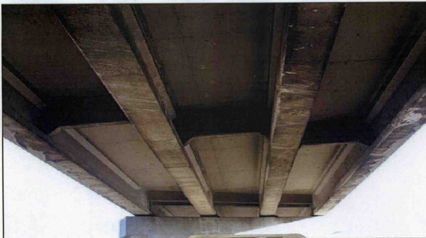
UNDERSIDE OF DECK
