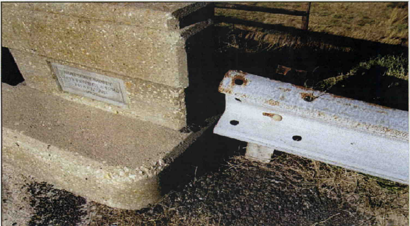
GUARDRAIL ATTACHMENT NORTHEAST CORNER
