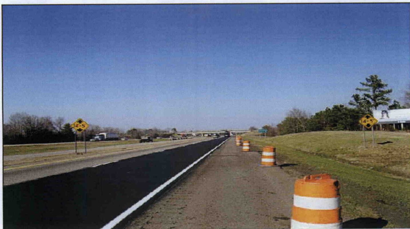
2 VERTICAL CLEARANCE SIGNS 14 FT.-5 IN. ON 95 NB 0.1 MI.S
