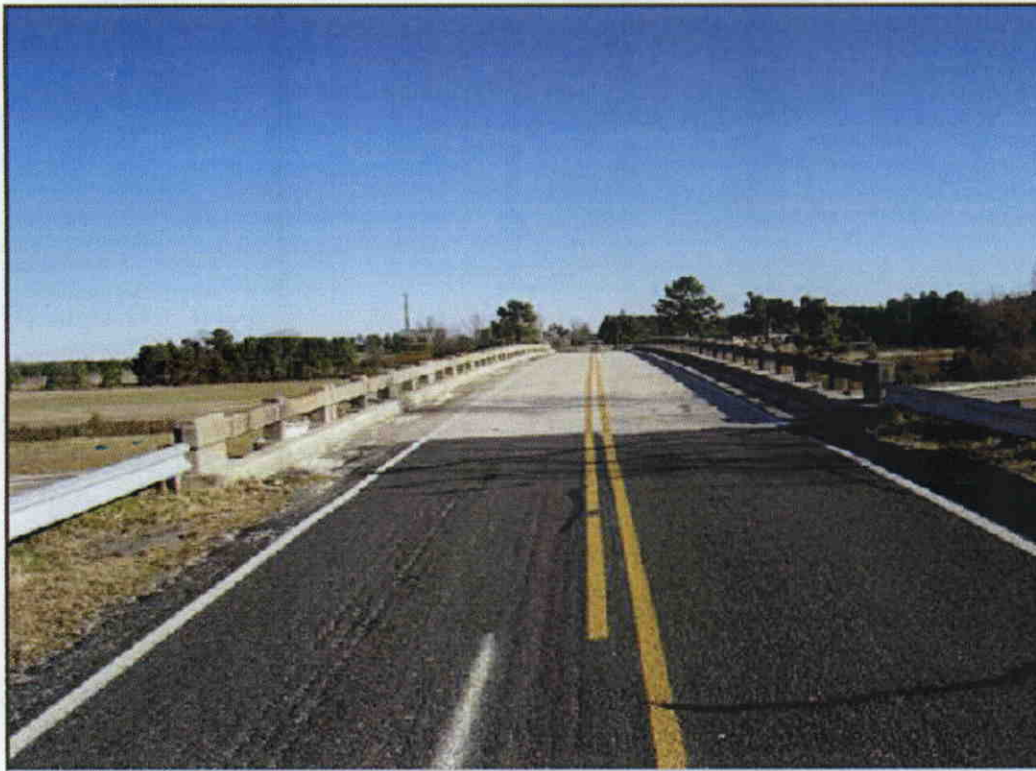
Photo Looking WEST APPROACH LOOKING EAST
