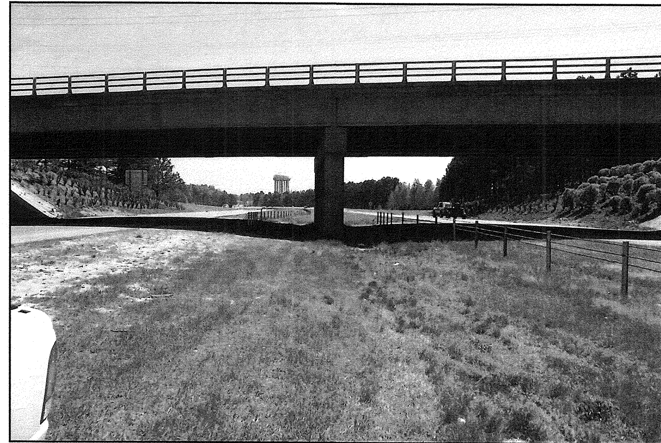
PHOTO 4: BENT 1, LOOKING SOUTH TOWARD BORING B1A
