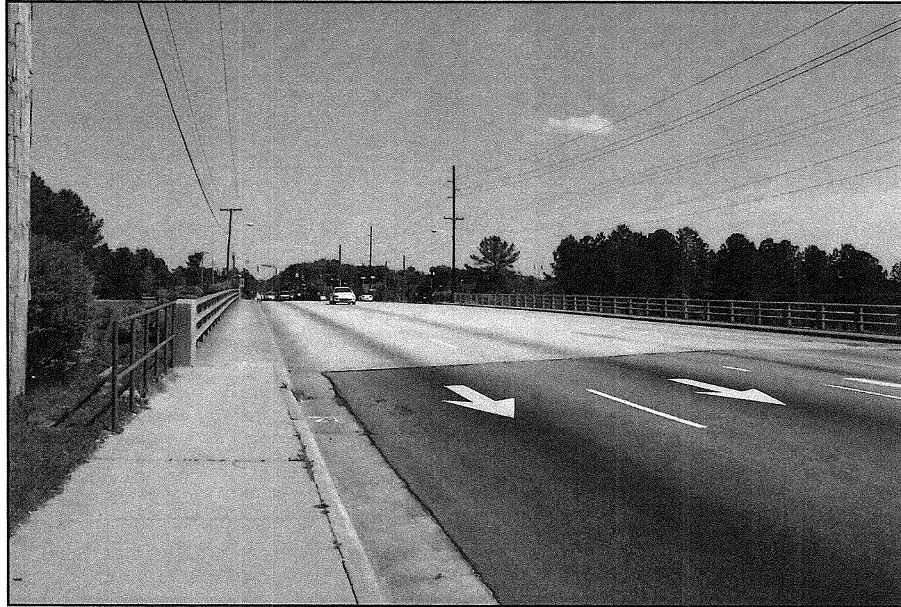
PHOTO 1: PROFILE 39' LEFT OF -L-, LOOKING UPSTATION
