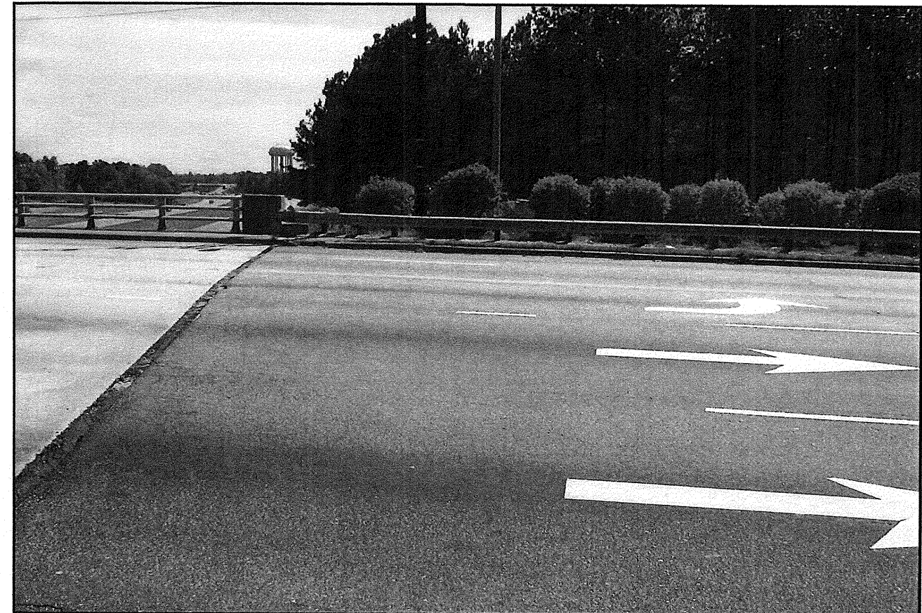
PHOTO 2: END BENT 1, LOOKING FROM LEFT TO RIGHT
