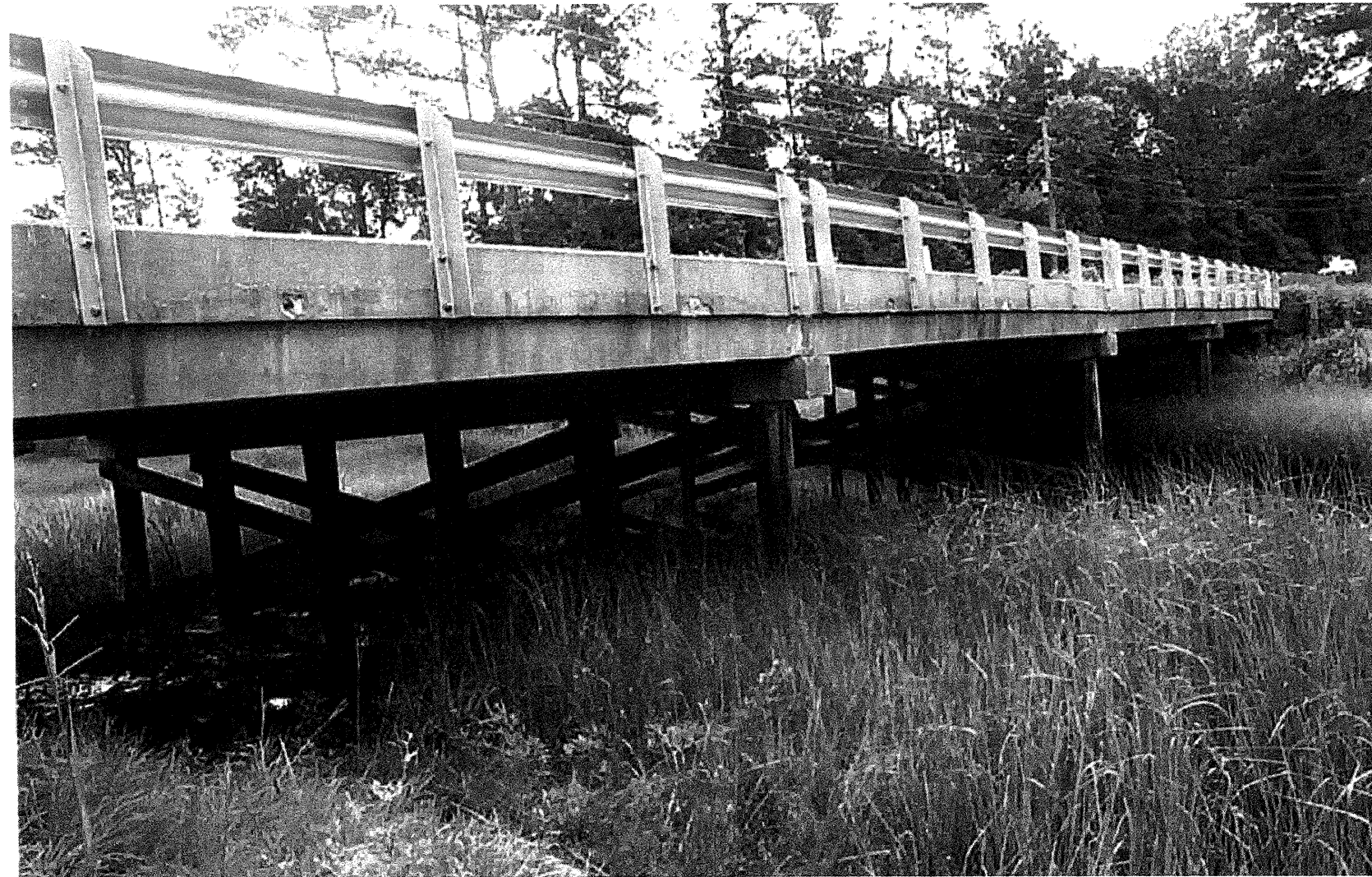
Looking Southeast Toward End Bent 1
