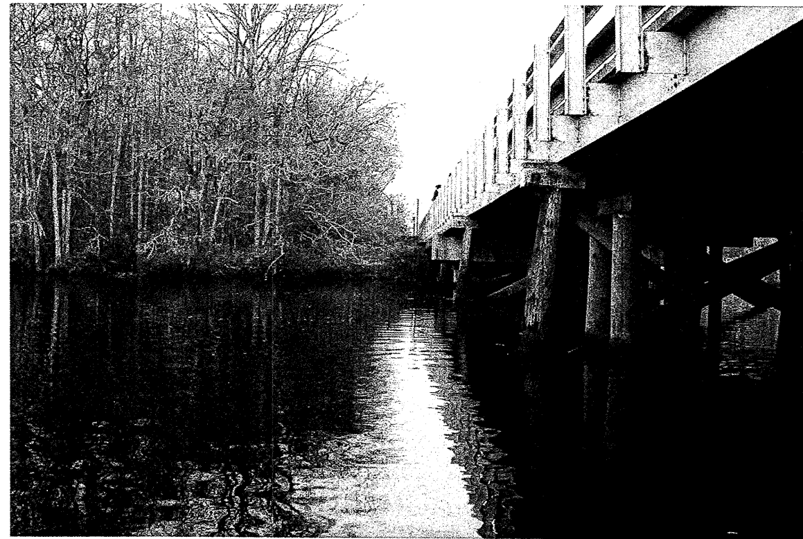
View looking down-station from Bent 6 along south side of bridge
