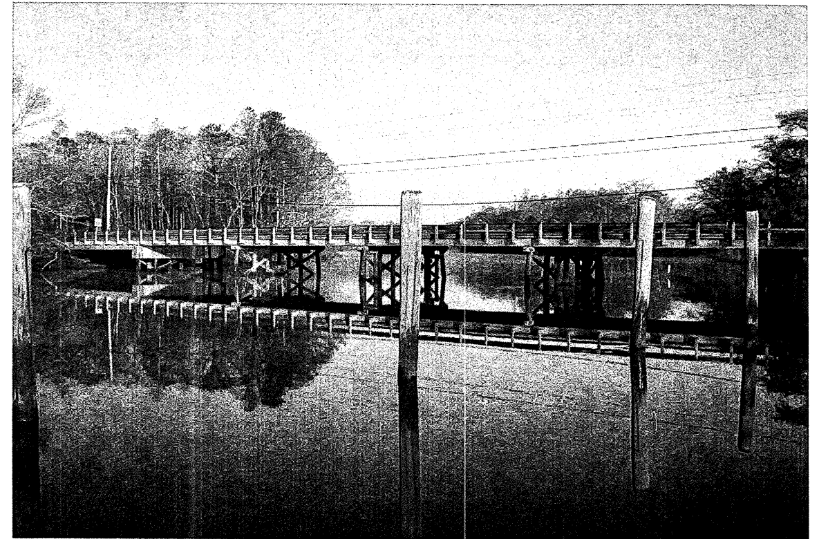
View looking north upstream
