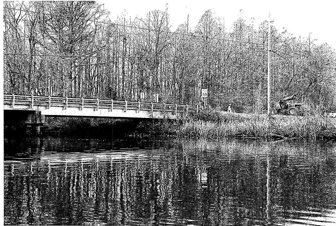
View looking south; drill rig at Bent 1
