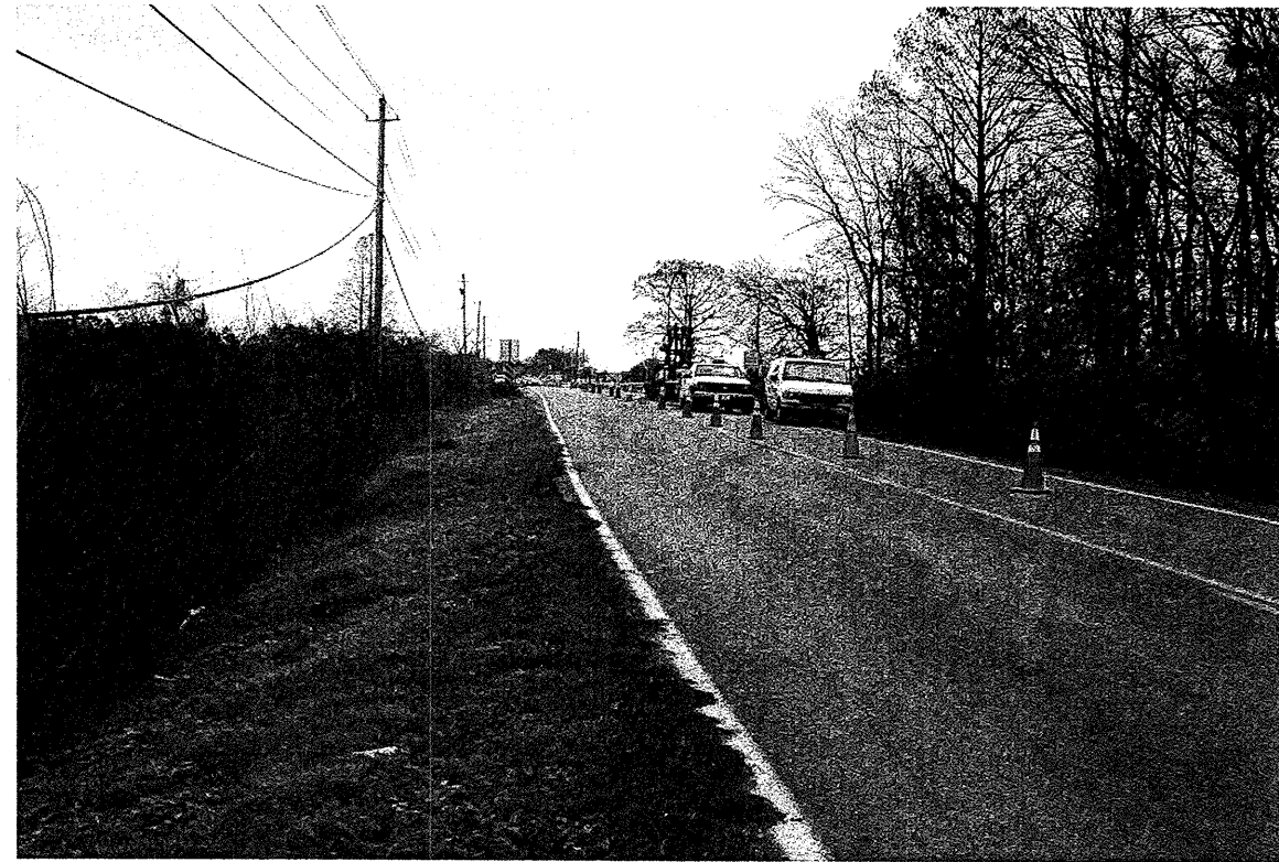
View looking east along approach to EB1
