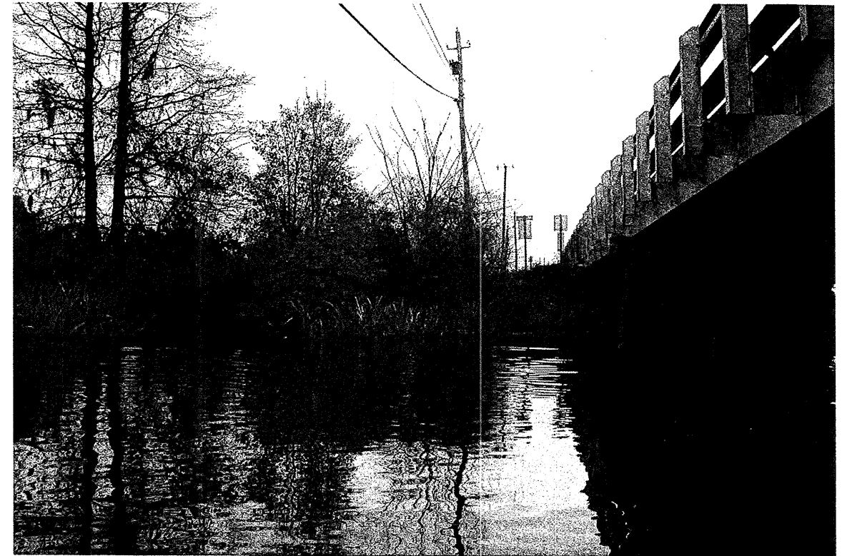
View looking up-station from Bent 6 along north side of bridge
