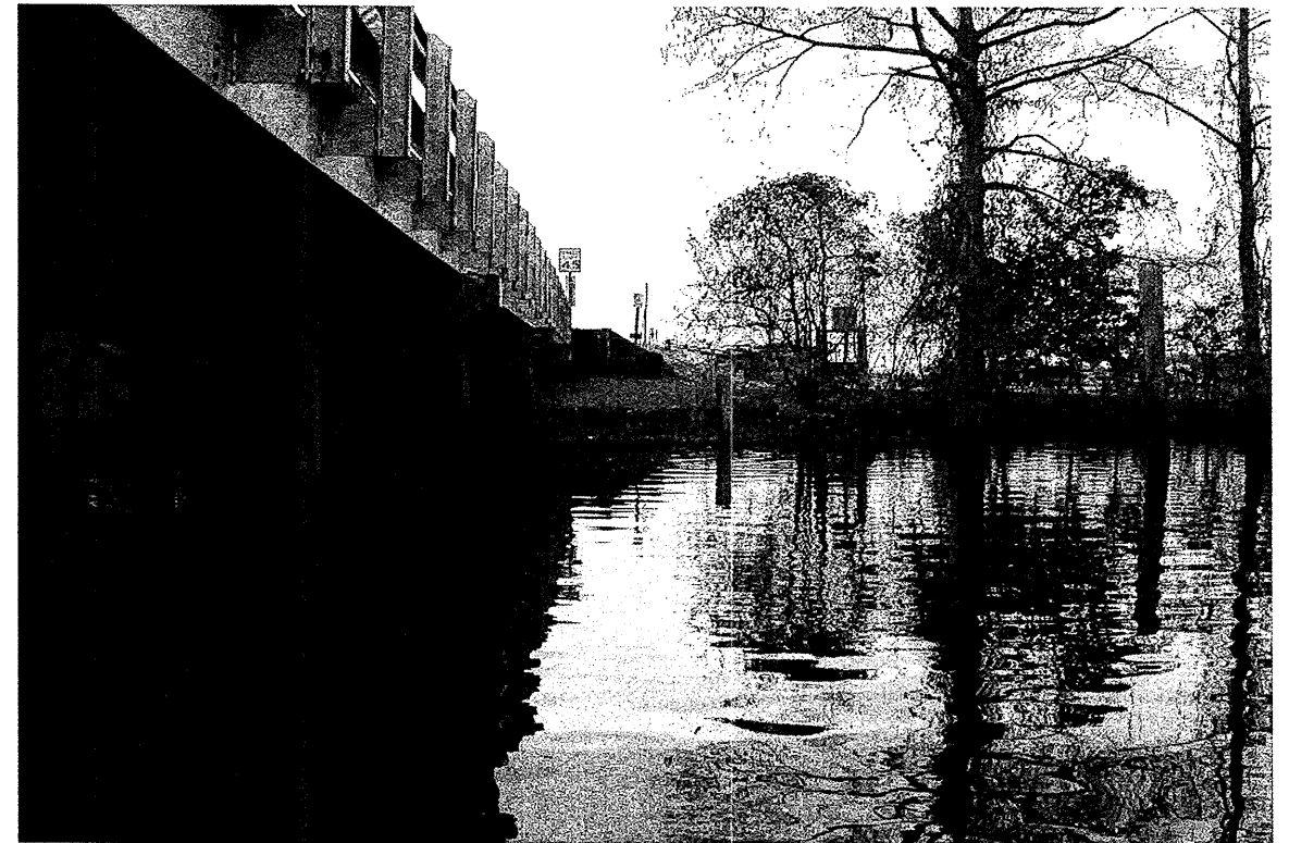
View looking up-station from Bent 6 along south side of bridge
