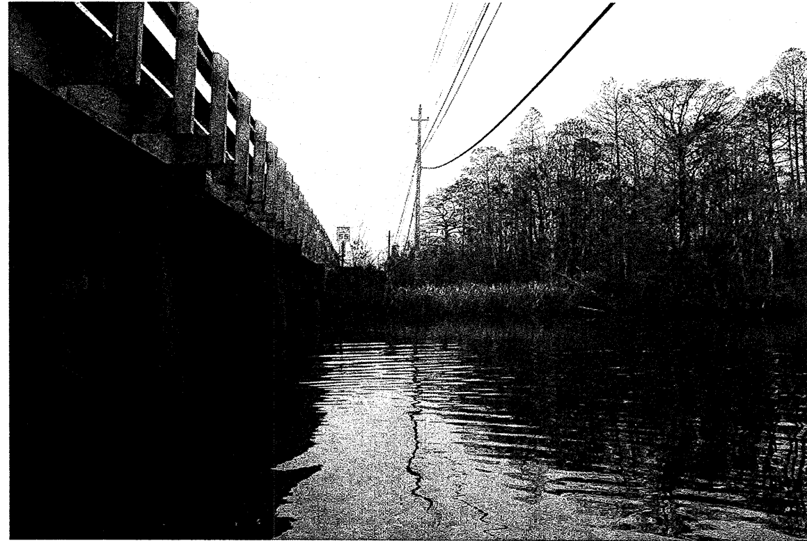
View looking down-station from Bent 6 along north side of bridge
