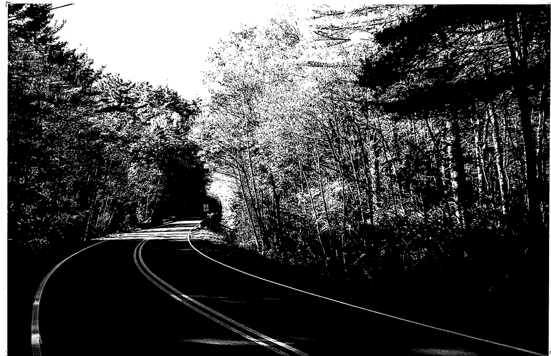
Figure 2. View looking back from Station 26+00, 40°RT.
