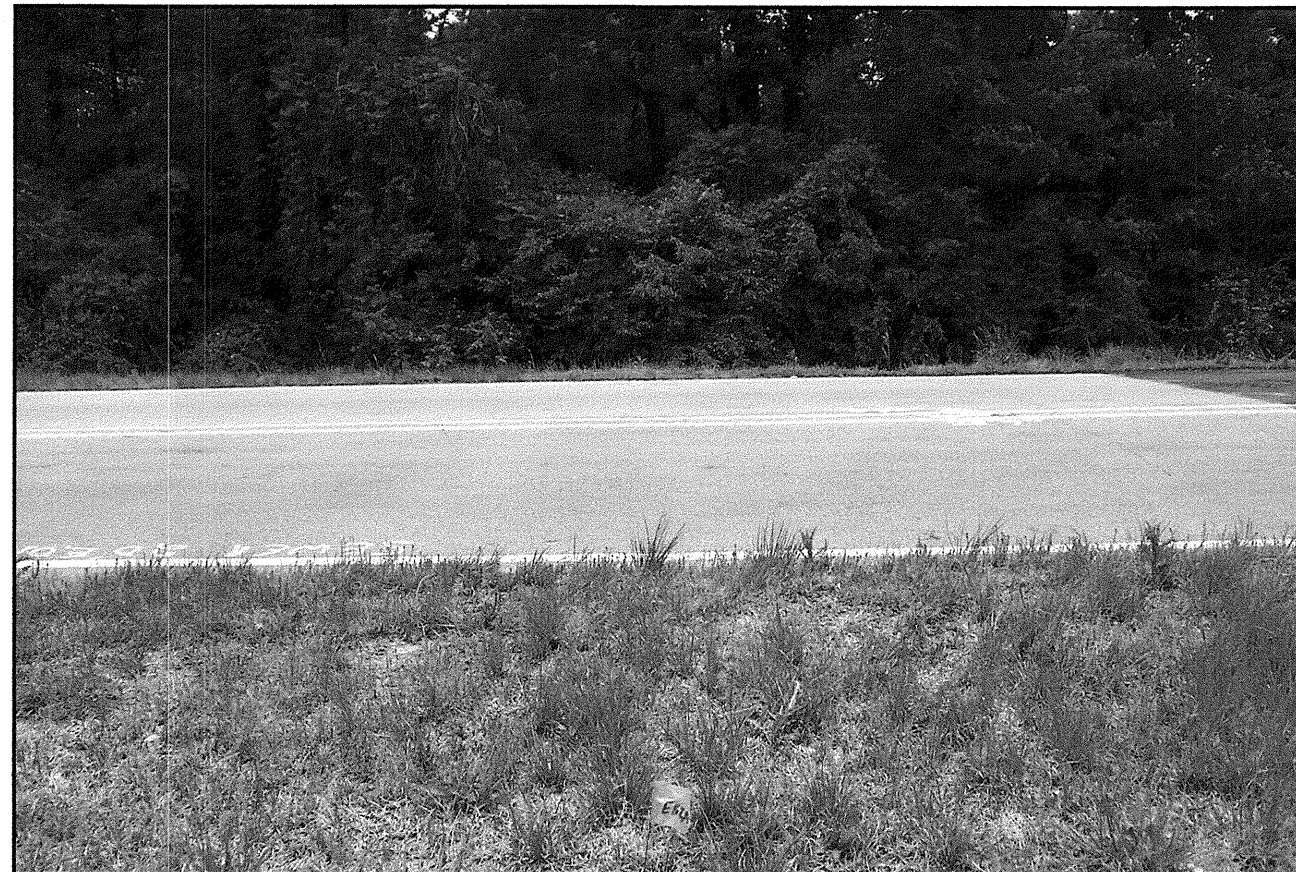
END BENT 2, LOOKING FROM LEFT TO RIGHT.
