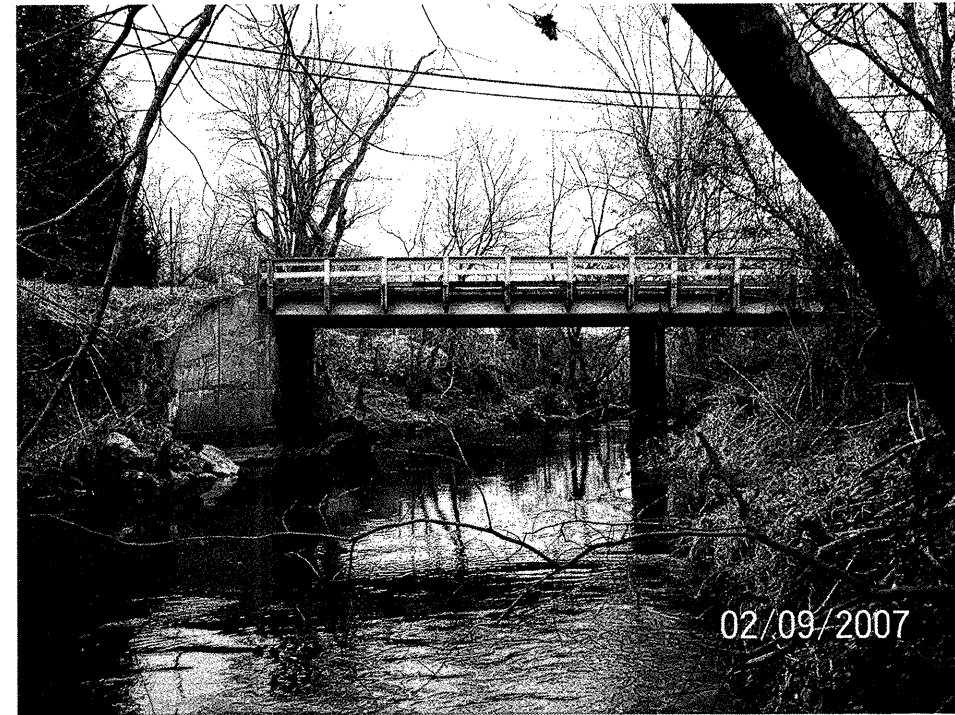
Photograph 11 – View of Existing Bridge Looking Upstream
