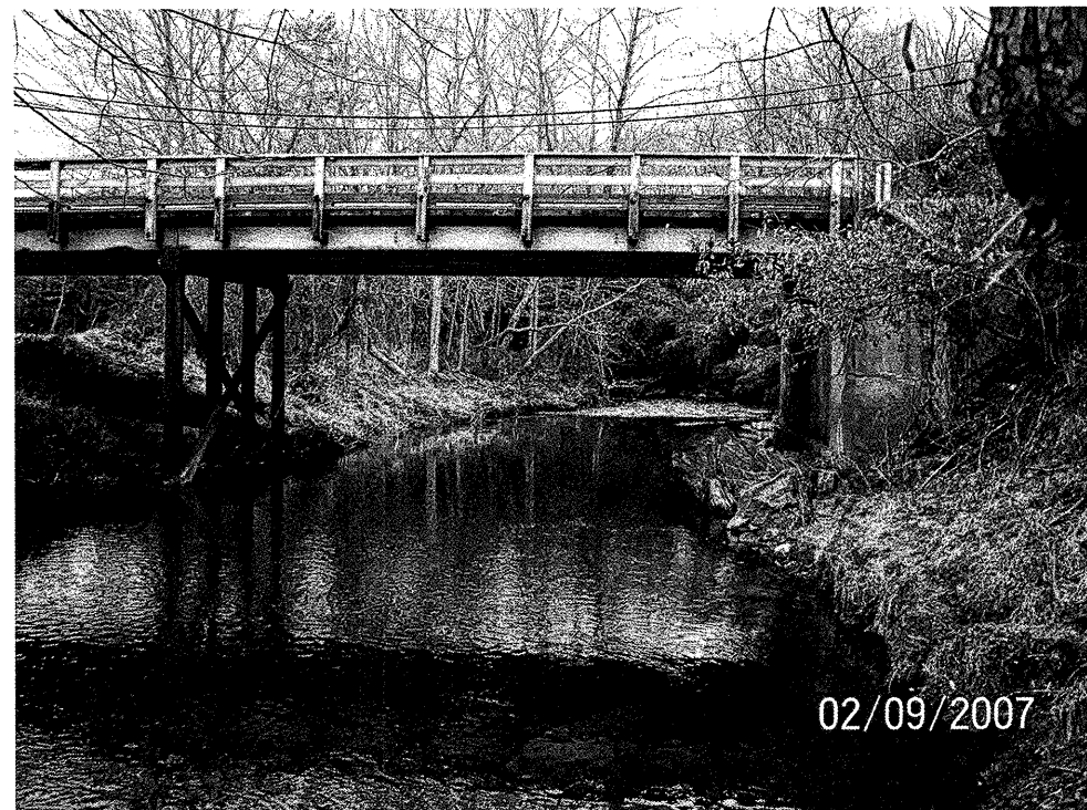
Photograph 10 – View of Existing Bridge Looking Downstream
