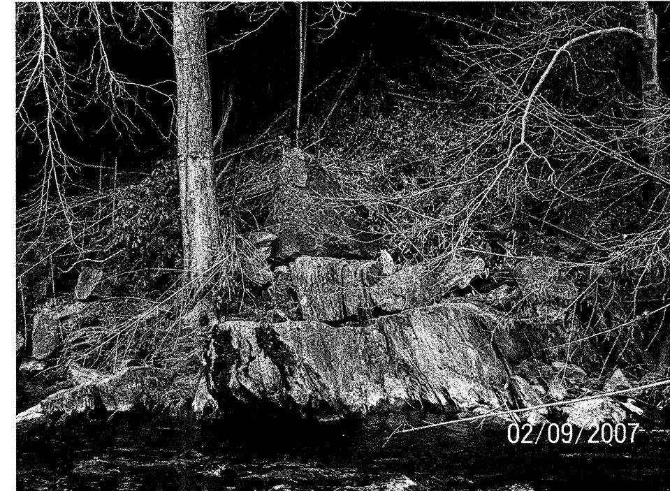
Photograph 8 – View of Rock Outcrop on North Bank at Proposed Location of New Bridge
