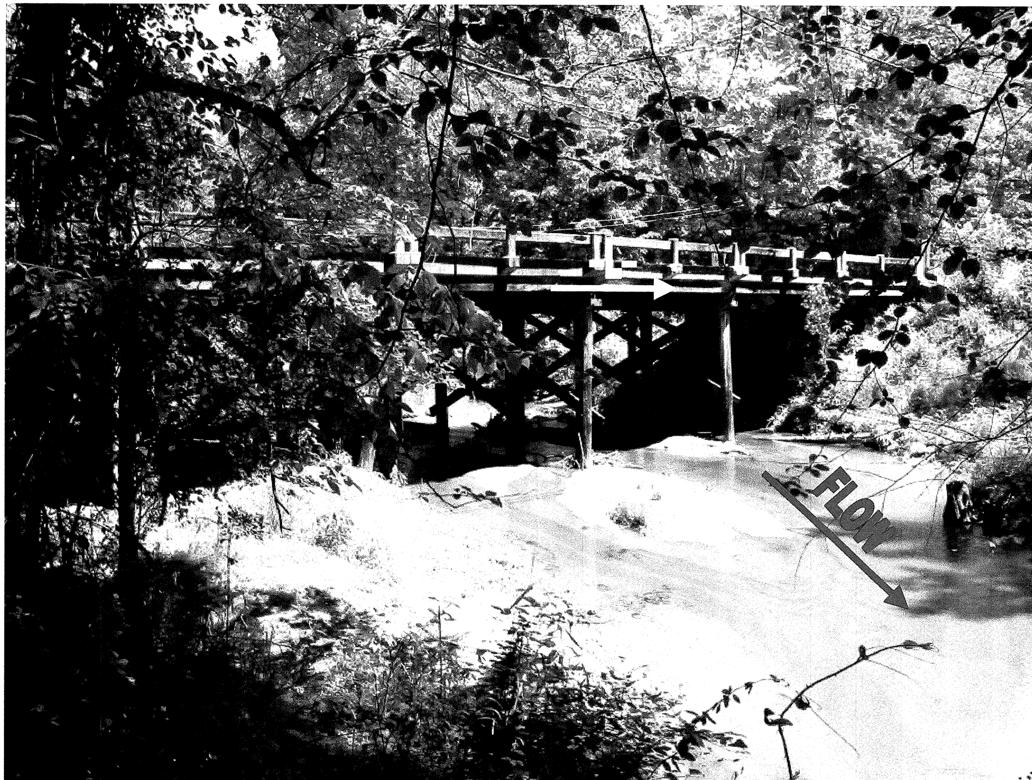
Looking North Towards End Bent 2
