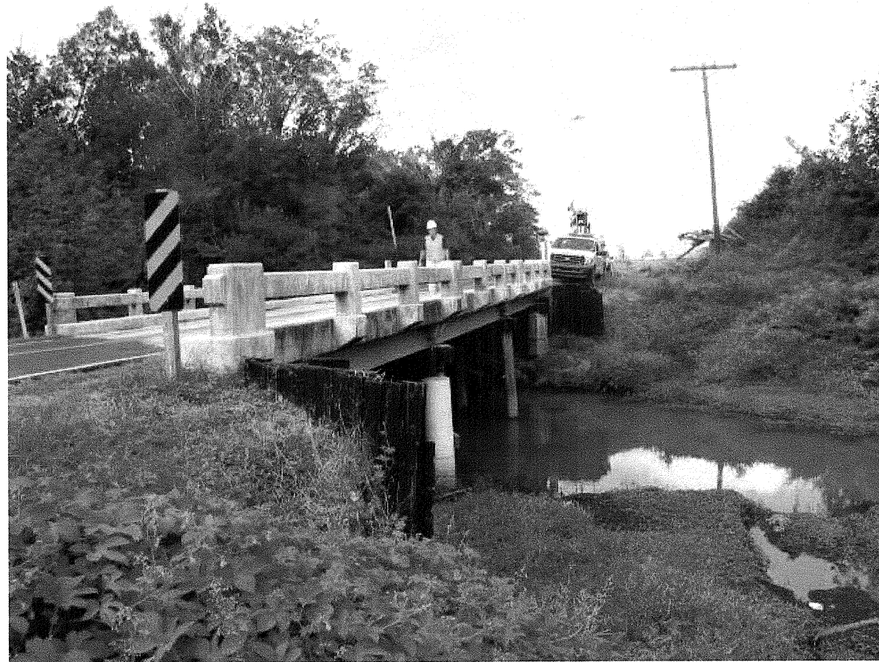
View Looking West Toward End Bent 1
