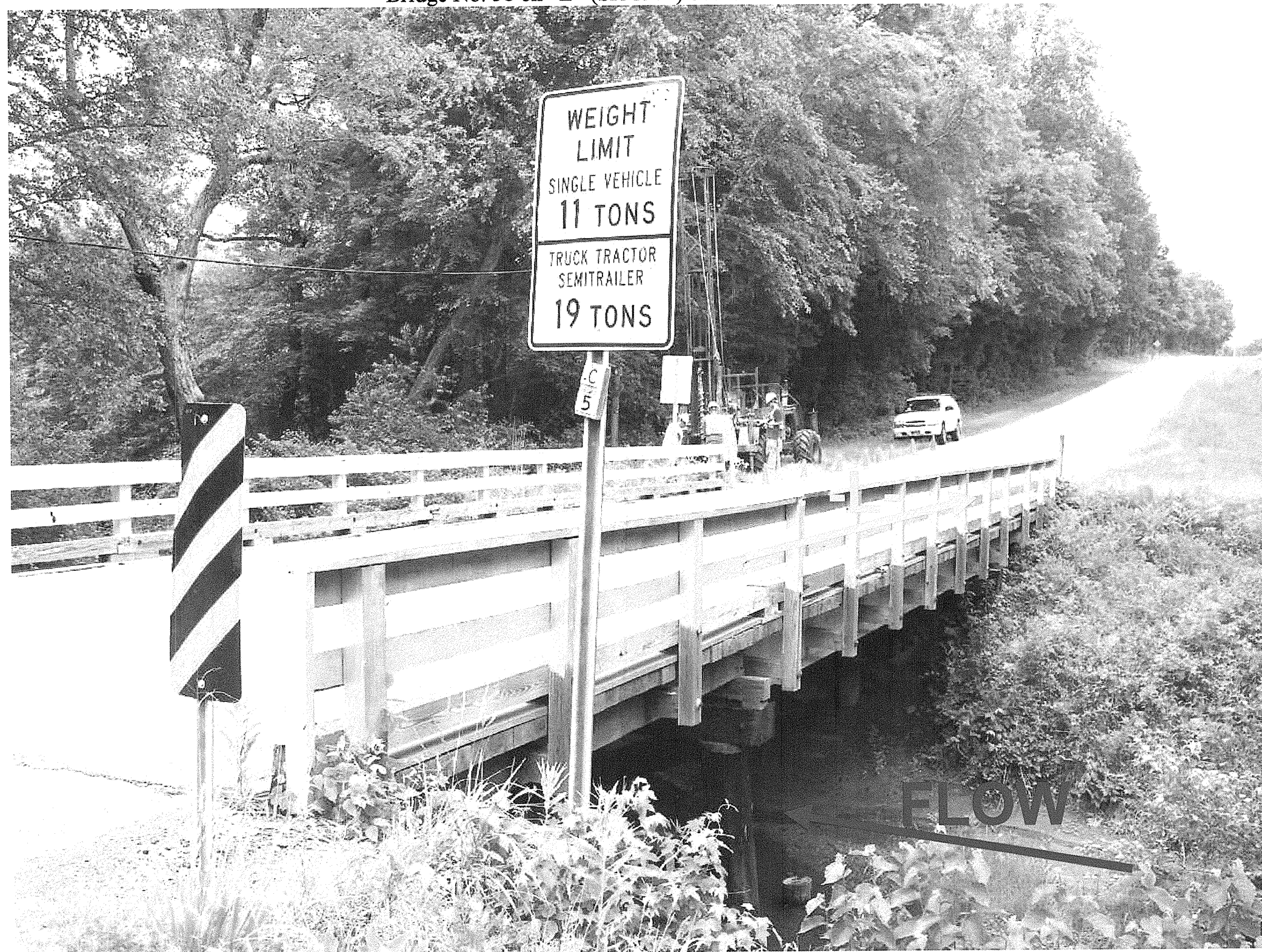
Looking Northeast Towards End Bent 2
