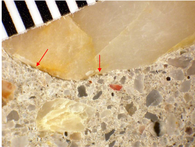
Figure 12. Adhesion crack partially surrounding coarse aggregate particle. Millimeter scale.
