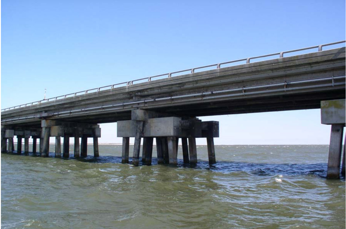
PHOTO 29: SUPPLEMENTAL PILES AND CAPS AT BENTS 173 THROUGH 186
