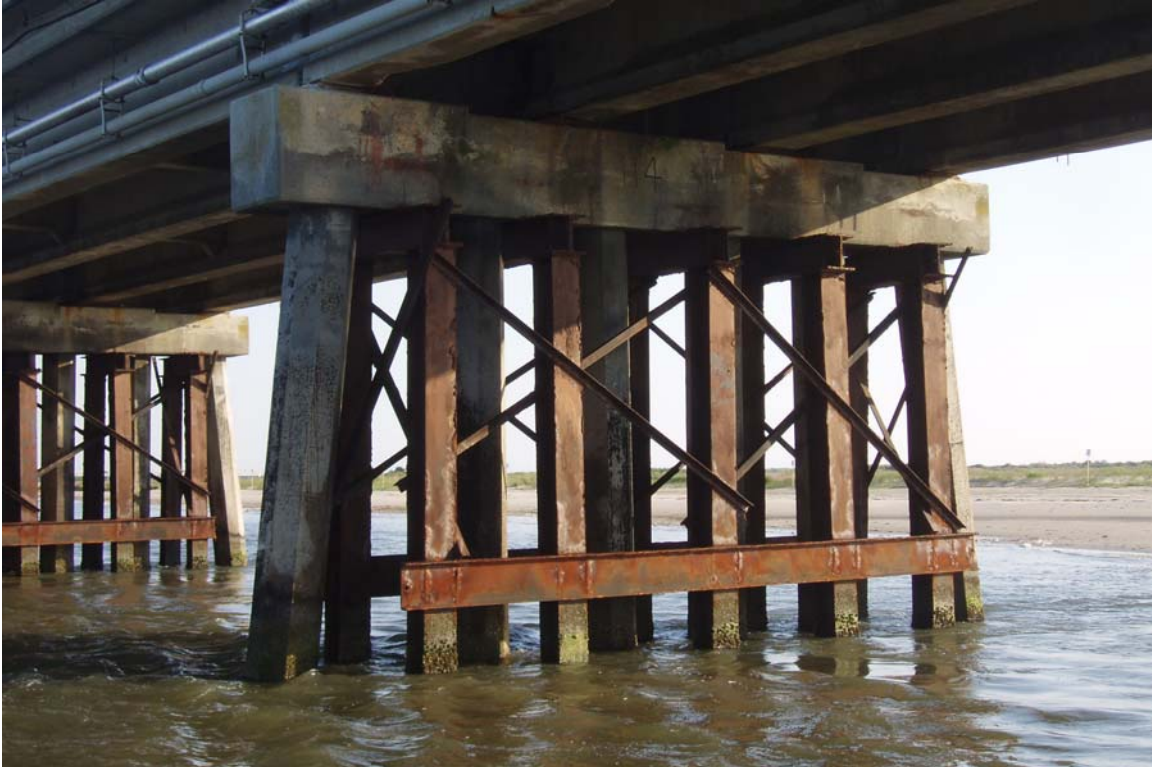
PHOTO 5: TYPICAL CONFIGURATION OF APPROACH BENT SUPPLEMENTED WITH H-PILES (BENT 115 SHOWN)
