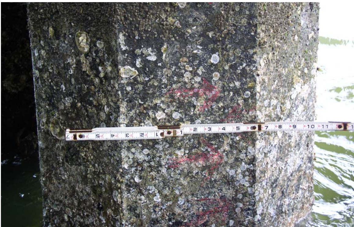
PHOTO 6: TYPICAL CRACKING IN CONCRETE PILE AT PILE 2 OF BENT 115
