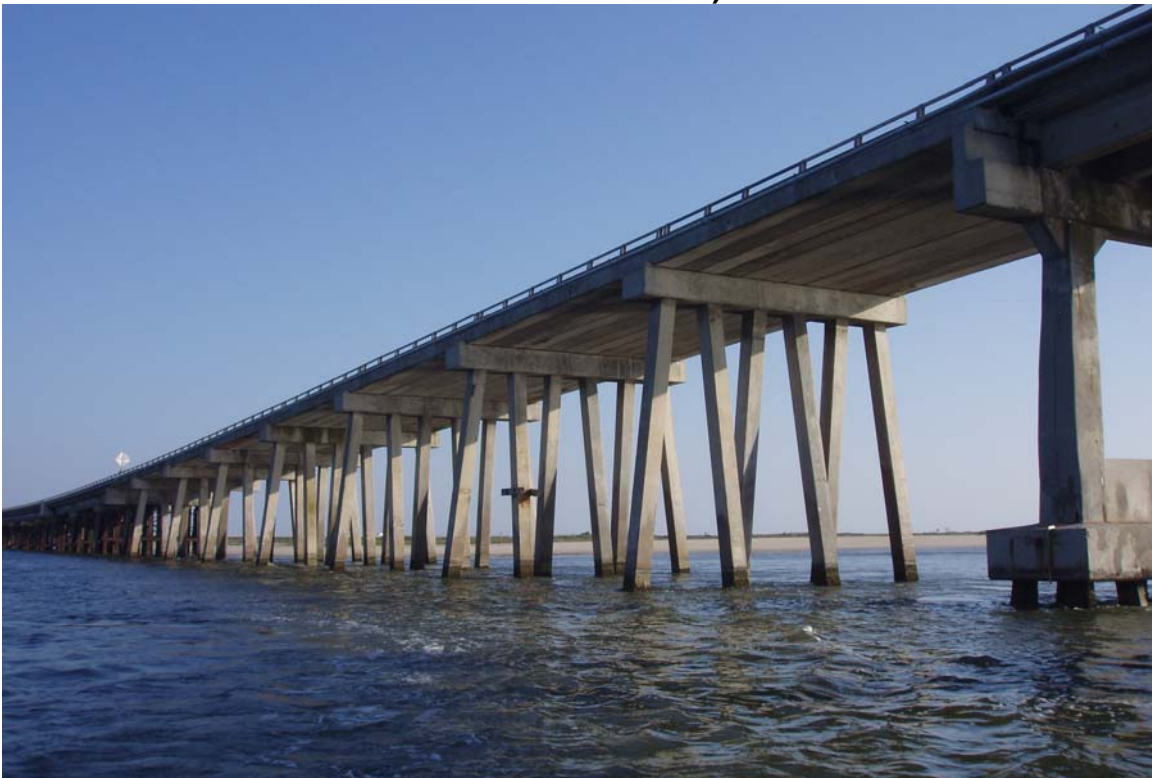
PHOTO 8: BENTS 124 THROUGH 128B, LOOKING NORTH
